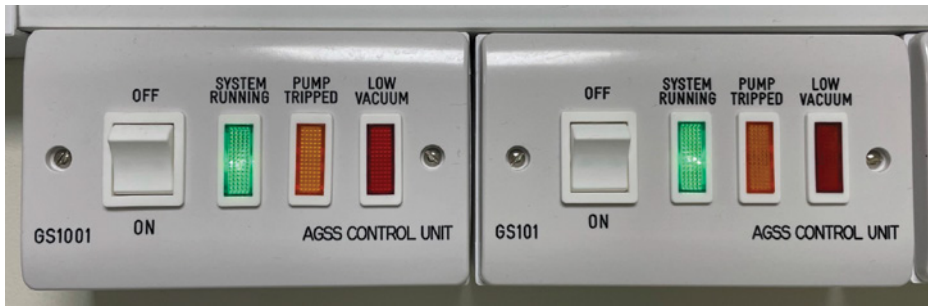
Figure 13.19 An AGSS local switch.
