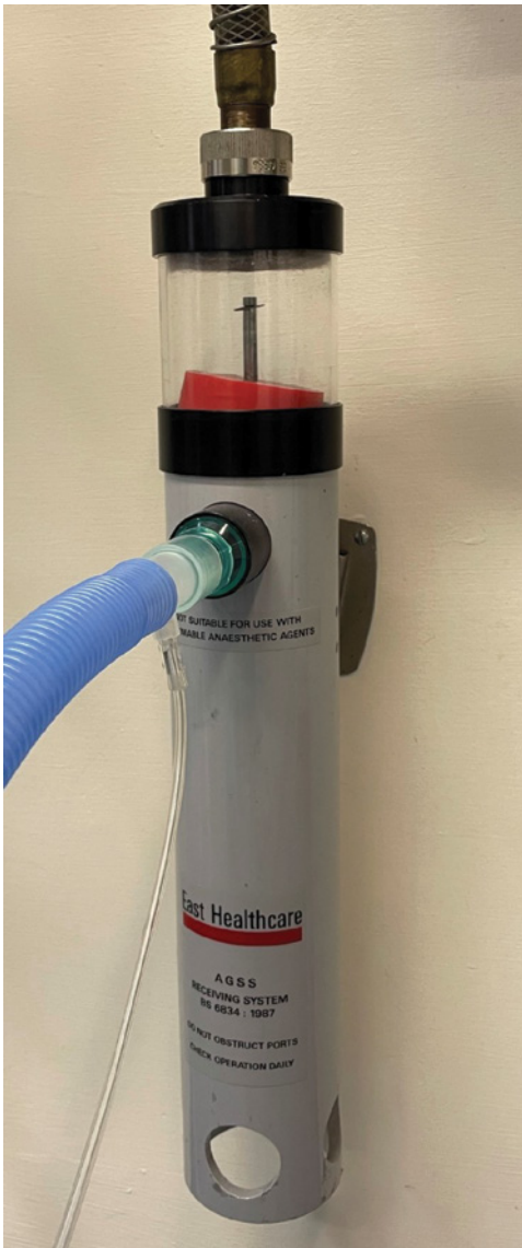
Figure 13.18 An air break receiver positioned between the patient (expiratory valve of the breathing system) and the AGSS wall outlet.
