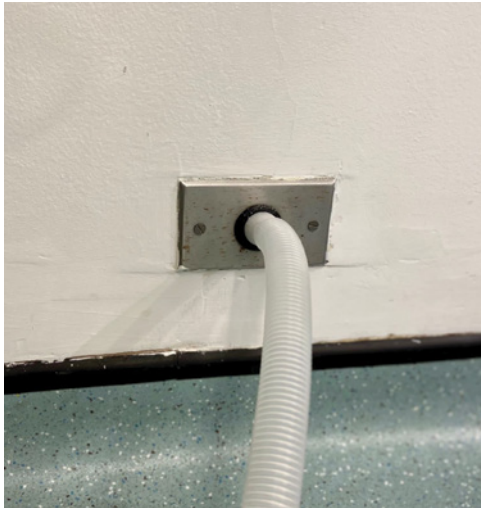
Figure 13.21 An outlet in the wall where anaesthesia gases can be vented. Photo credit: Louise Northway.
