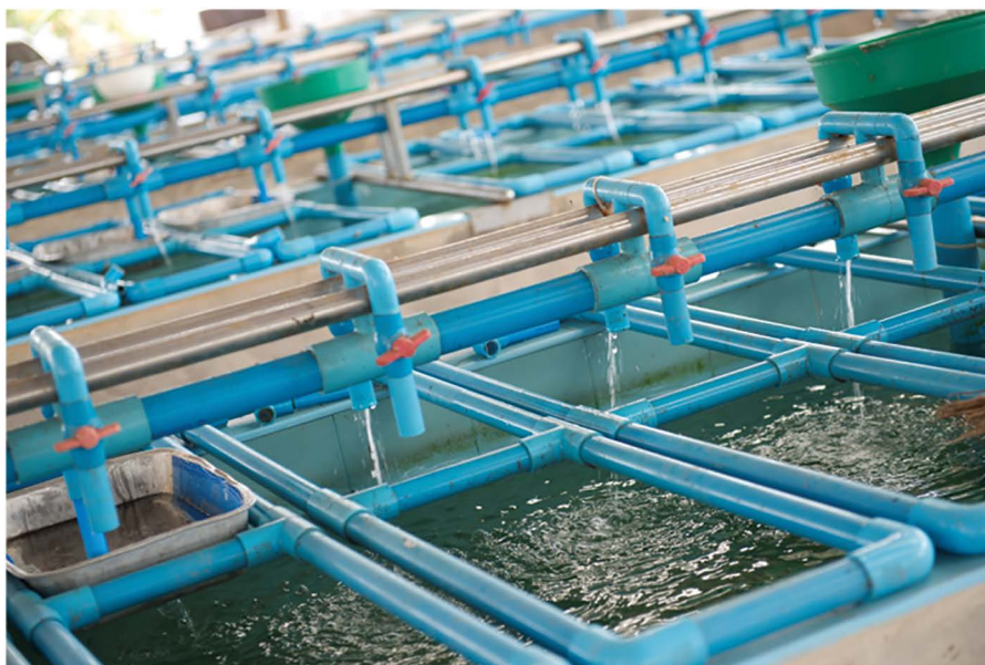
Fig. 11.5. Building biosecurity into the infrastructure of production sites. The design of a site should minimize cross-contamination between different sections; permit the management/treatment of water flow through the site; and permit each production unit to be effectively disinfected on a routine basis. (Image courtesy of Fish Vet Group Asia, Benchmark.)
