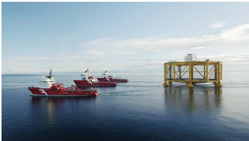
Fig. 11.7. Owned and operated by SalMar, Ocean Farm 1 is the first salmon farm designed and built for exposed operation, with a novel design that combines solutions from aquaculture and the offshore industry. ( https://www.dnv.com/news/ocean-farm-1-receives-first-ever-offshore-fish-farming-class-certificate-from-dnv-gl-165626 , accessed 12 January 2023.)
