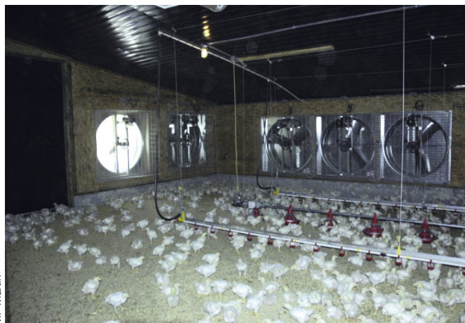
Fig.2.12: Ventilation maintaining good air quality and litter conditions.
