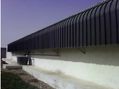
Fig.7.17 & 7.18: Cooling pad. Exterior appearance with partial recovery of water and interior view.
