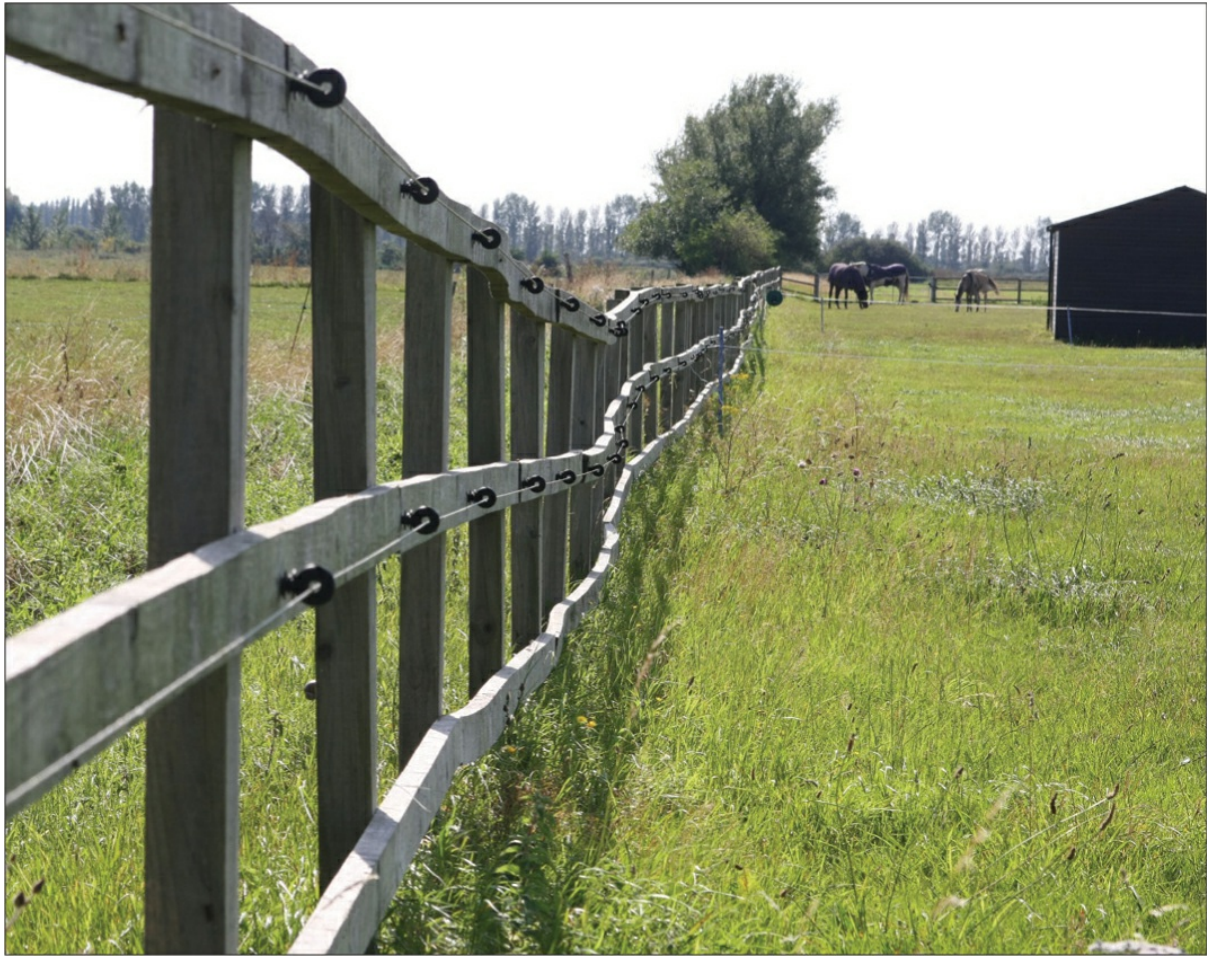
Post and rail fencing with offset electric wire.
