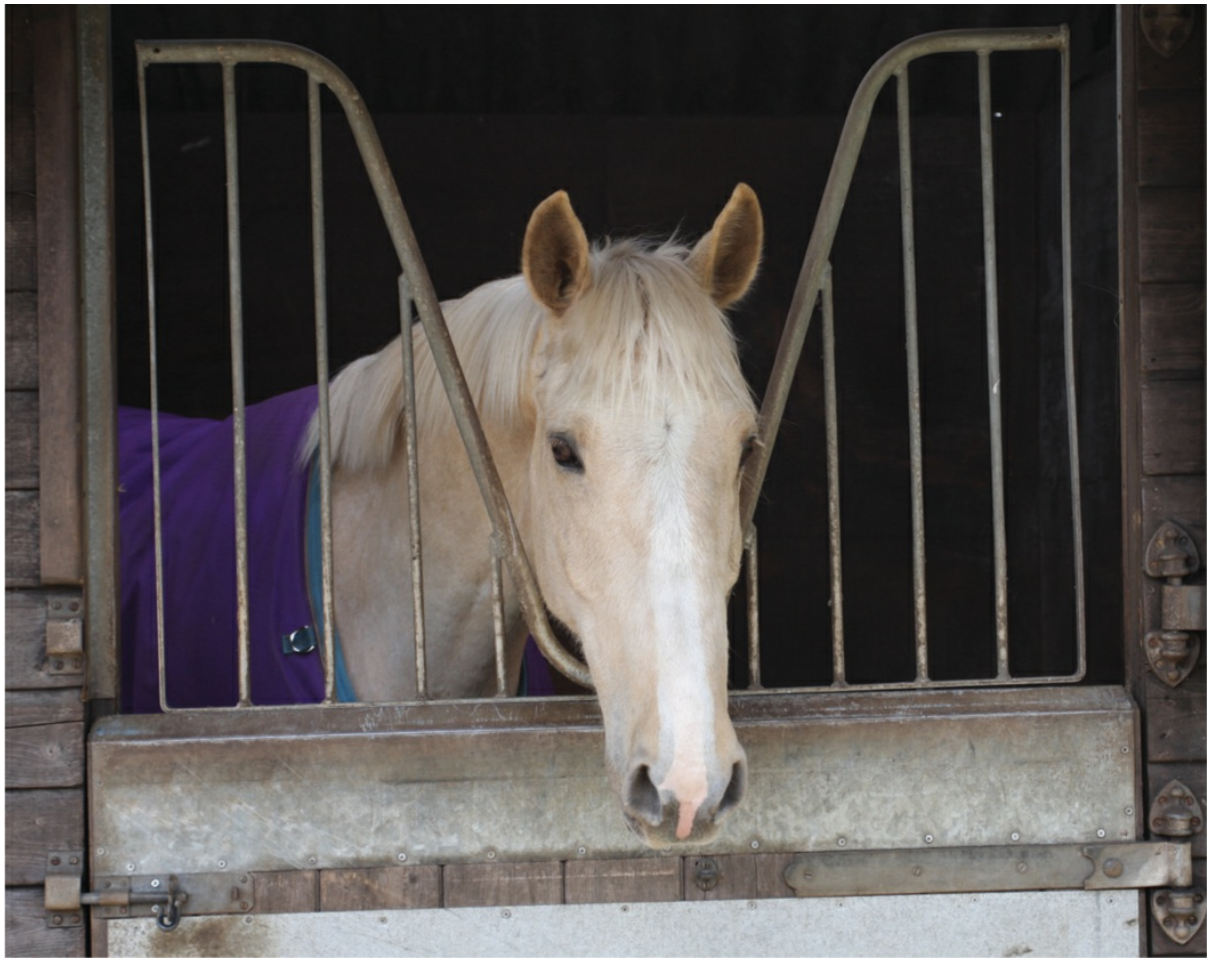
V-shape grilles discourage horses from trying to jump over a stable door.
