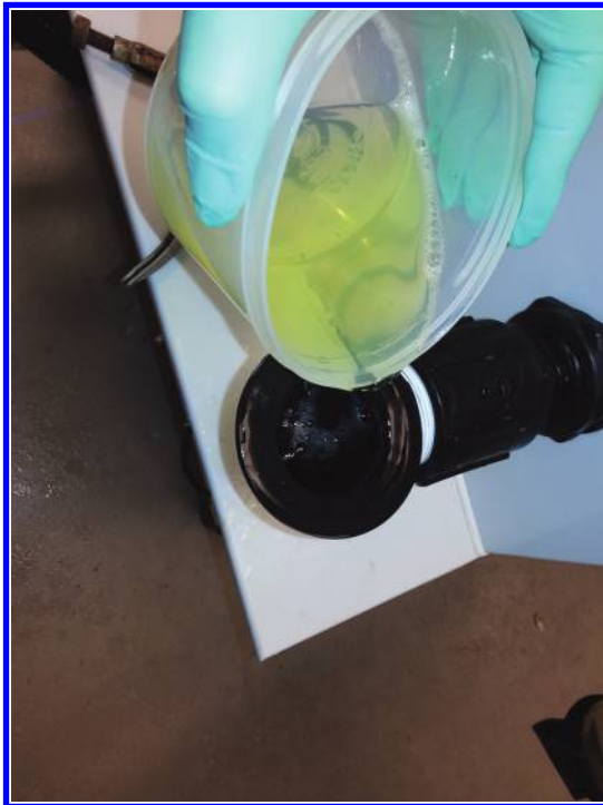
Figure 6.73 Fill fitting assembly with sterilant.
