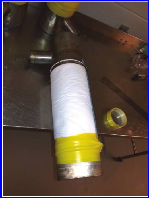
Figure 6.7 Cover the clamp with nylon tape.
