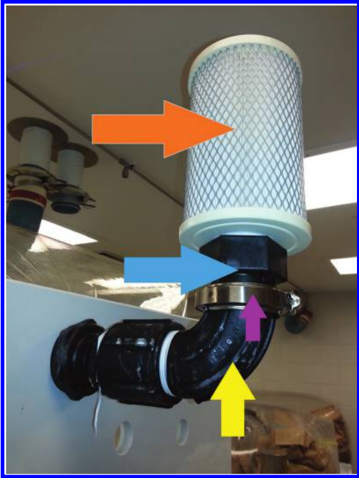
Figure 6.76 Appearance of the filter assembly with filter installed: The filter (orange arrow) is installed onto the filter adapter (blue arrow) and secured with a clamp (purple arrow). The yellow arrow indicates the previously installed fitting assembly.
