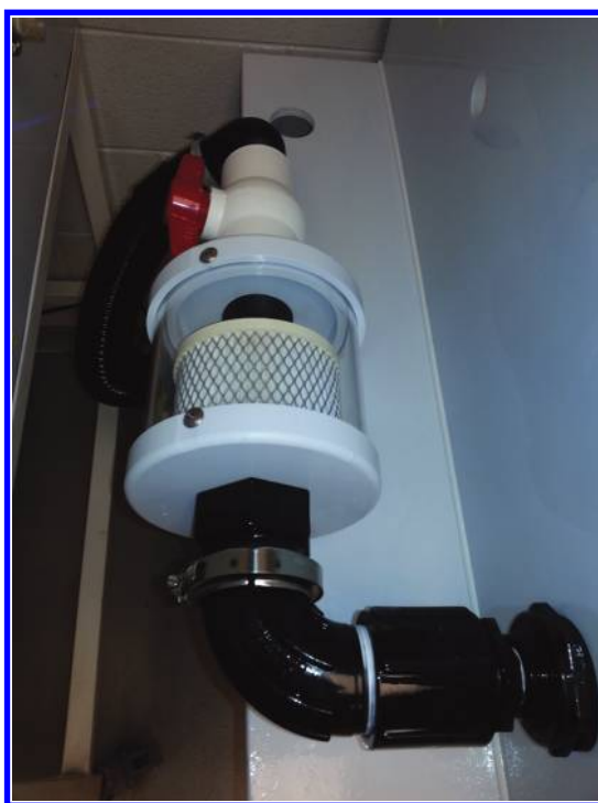
Figure 6.90 The final horizontal position of the intake filter connected to the air supply.
