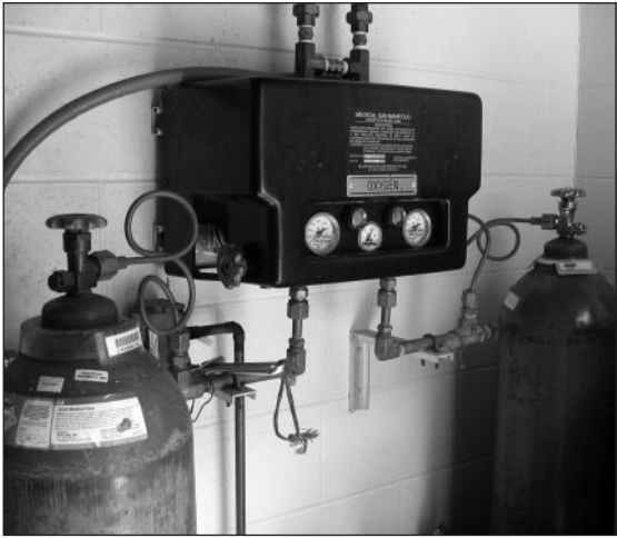
Figure 3-4 Bank of 2 oxygen tanks connected to manifold for central supply. One tank is open to system with the other tank in reserve.
