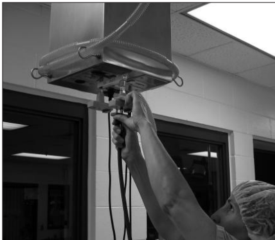
Figure 3-8B Rigid Ceiling column with Fresh Gas Pressure Outlets. Veterinary Teaching Hospital, Michigan State University
