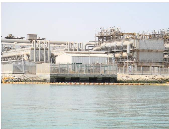
Figure 4. Sitra power and desalination plant discharges brine waste water that associated with high levels of salinity and temperature.
