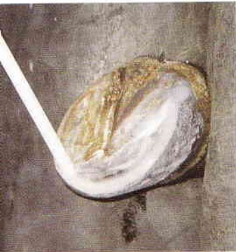
FIGURE 13: The polymer is applied along the outer wall and into the sulcus.
