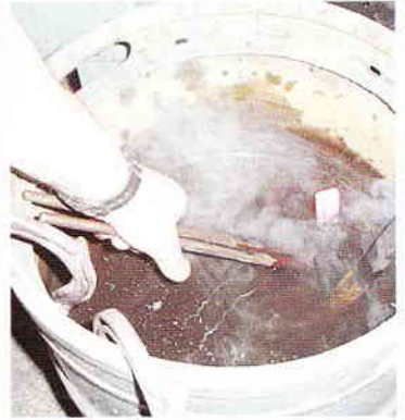
FIGURE 33: Take a short heat approximately 25 mm (1 inch) from the end before jumping up the branch.
