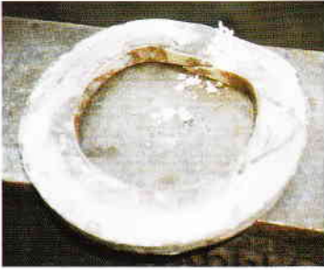
FIGURE 25: The aluminium coil and flux is placed over the scarf prior to welding.
