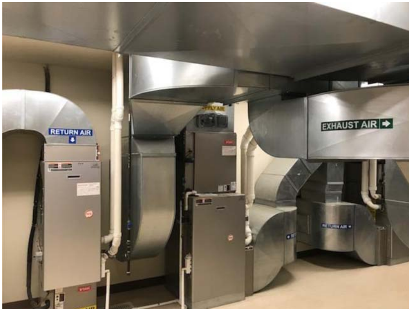
Figure 8.3 RCAC air handling system.
