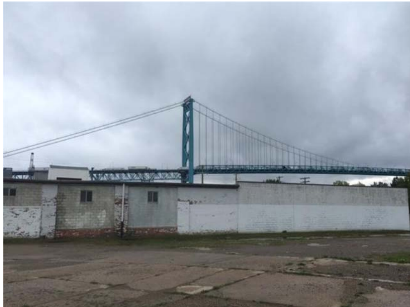
Figure 7.2 Old DACC facility.
