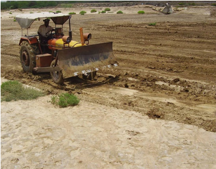
Renovating the pond (using tractor dozer)
