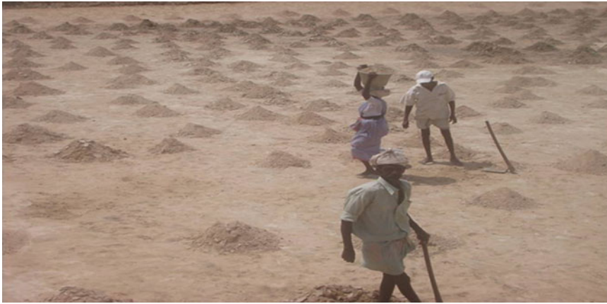
Scraping the pond bottom (using man power)
