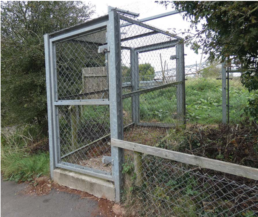
Fig. C4 Containment: Double door entry system.
