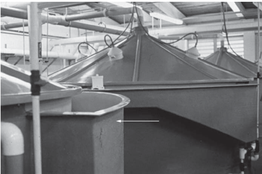
Fig. 6.19. An egg-collecting box on the side of a red drum spawning tank (the arrow points to the box).
