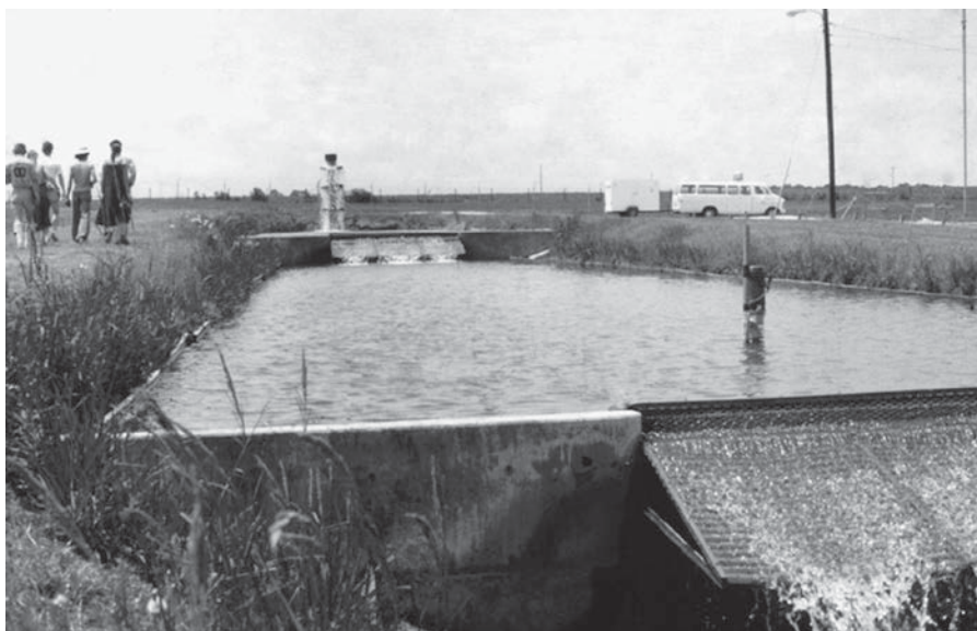
Fig. 3.20. A series of raceways with splashboards between them for aeration. Note that at the top of the series there is a splash tower that aerates the water entering the first raceway in the series.
