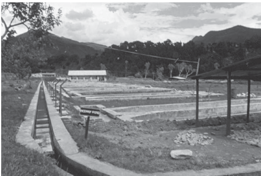
Fig. 3.18. Trout raceways in Nepal. Note the presence of an open channel for inflow water.
