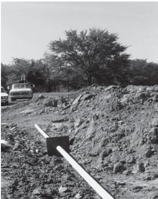
Fig. 3.12. The metal antiseep collar set in place immediately prior to having the levee built over it.
