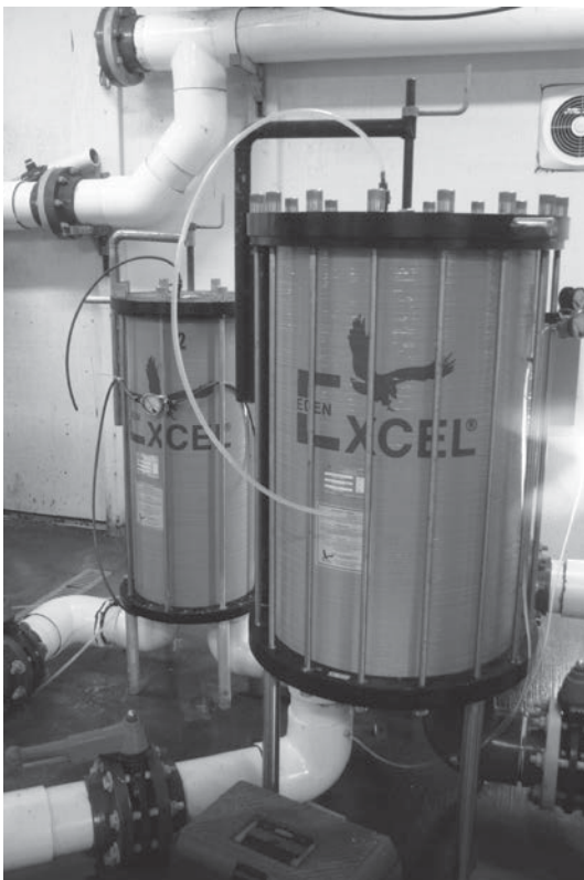
Fig. 3.27. Cartridge filters are sometimes used to remove very fine particles from culture water.
