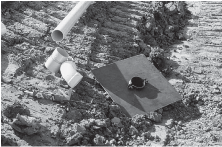
Fig. 3.11. A metal antiseep collar and some of the PVC components prior to being assembled.
