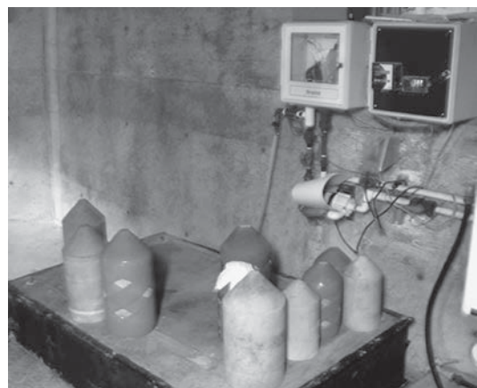
Fig. 3.45. Pigs of various sizes, behind the scenes at a large public aquarium, are pushed through incoming water pipes periodically to scrape out the fouling organisms.
