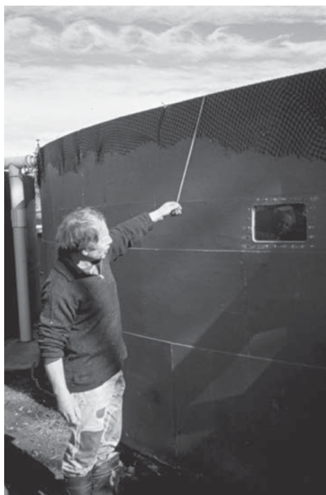
Fig. 3.21. A large circular production tank in New Zealand. The tank is somewhat unique in that it was constructed of plywood instead of plastic or fibreglass.
