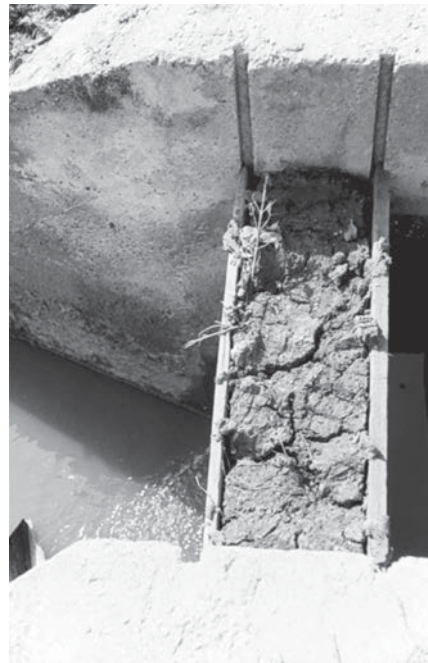
Fig. 3.13. A portion of a pond drain kettle in a Malaysian shrimp pond showing two sets of baffle boards with dirt between them to reduce seepage.
