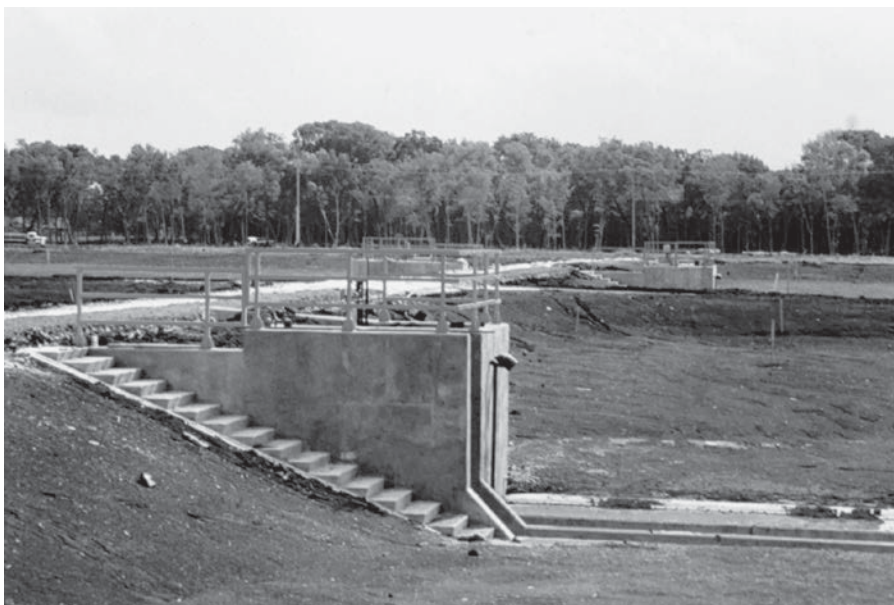
Fig. 3.15. This multifunction kettle at a state fish hatchery in Texas, USA, features an inflow line, drain valve, stairway and catch basin.
