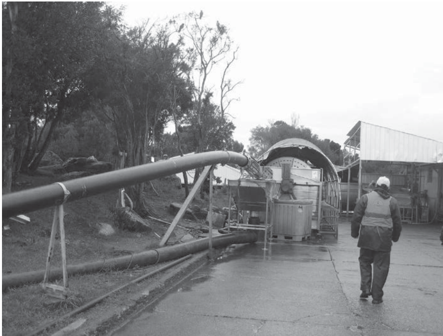
Fig. 9.16. The chilling tank referred to in Fig. 9.15 is located at the end of the pipeline leading from the fish pump.
