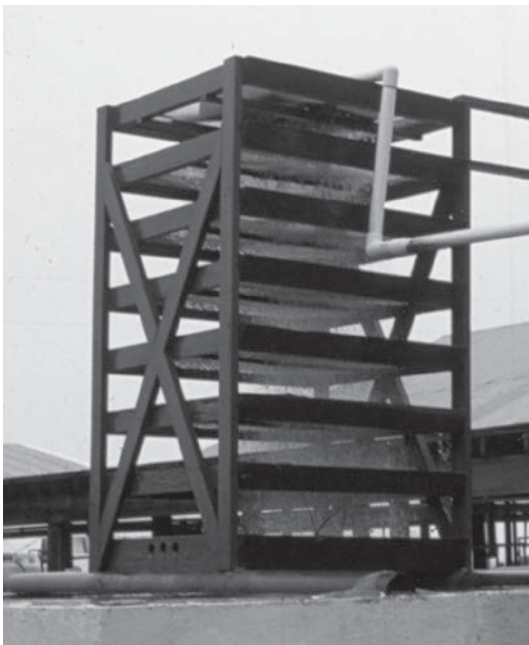
Fig. 2.3. An aeration tower such as this is basically a stack of screen-bottomed boxes that break up inflowing water to increase the amount of area exposed to the atmosphere. This approach can oxidize ferrous iron to ferric hydroxide, drive off carbon dioxide and hydrogen sulfide, and saturate the water with oxygen.
