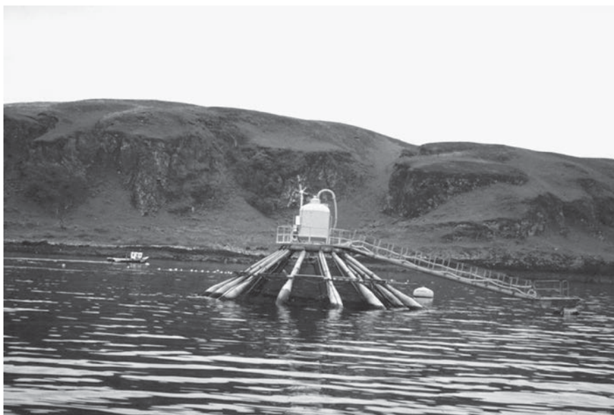
Fig. 3.35. The open ocean net pen system shown here was a design developed in Scotland that could withstand 6 m waves. While the one shown is near the shore, the fetch of the wind was so long that such waves were sometimes experienced. The long legs are partially filled with water to submerge part of the system. The large bin at the top contains feed that is released automatically. The bin holds several days worth of feed.
