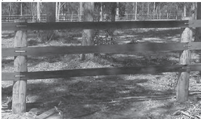
Figure 4. A post-and-rail fence, 1.3 m high (courtesy Jane Myers).
