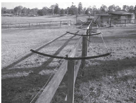
Figure 8. An offset electric wire using poly pipe outriggers (courtesy of Jane Myers).
