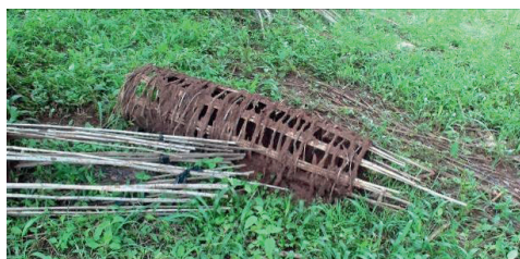
Figure 7.19 Starting to apply the mud outer casing
