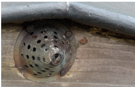
Fig 11.54 The hives' ventilation blocked with spiders and debris reducing air flow in the hive
