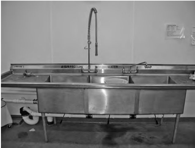
FIG. 5 Three-compartment stainless steel sink installed in food production area for hand washing and sanitizing of utensils and small equipment.
