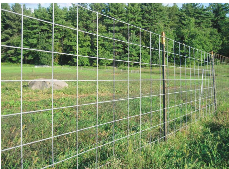
Cattle panels attached to T-posts make a sturdy fence, particularly for younger animals.
