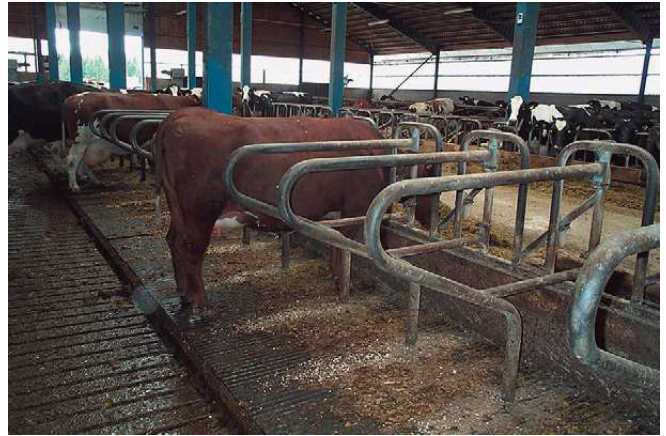
Figure 6-16 A spacious barn with a central feed truck alley between two rows of feed stalls with individual stall partitions and rubber flooring. (Courtesy of C Bergsten)
