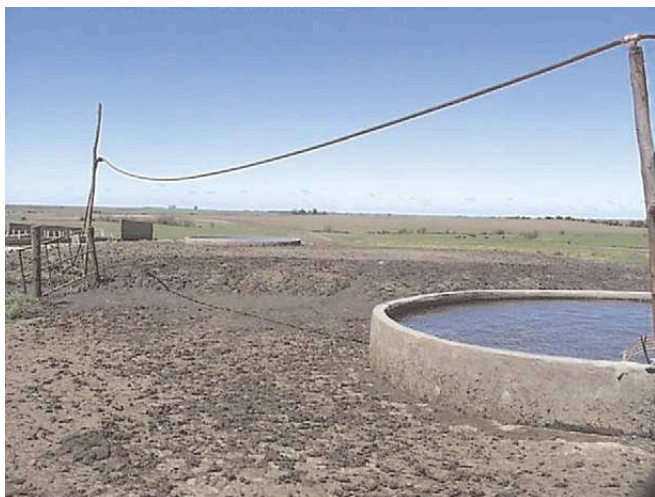
Figure 9-1 Although this watering station provides good perimeter access, it is too low to the ground; the perimeter around is very muddy and should have a concrete apron. (Courtesy of R Acuña)
