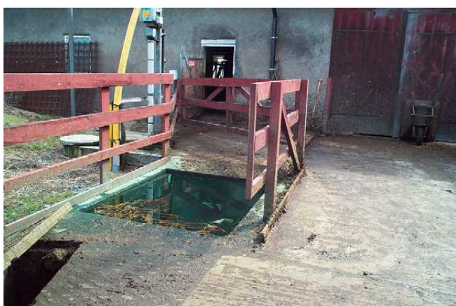
Figure 14-31 This foot bath is located in the open and is not sufficiently long to provide good service. (Courtesy of C Bergsten)
