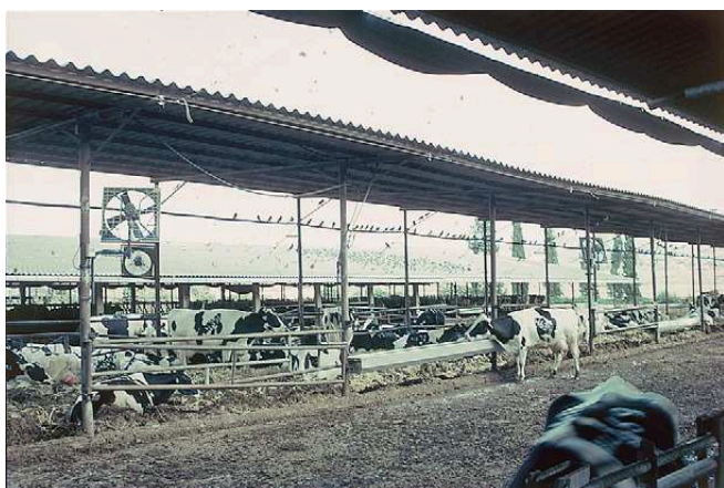
Figure 6-19 In tropical climates (such as this yard for dairy cows in Israel) barns have high roofs, cooling fans and in some cases water sprays to help lower the body temperature of the cows.
