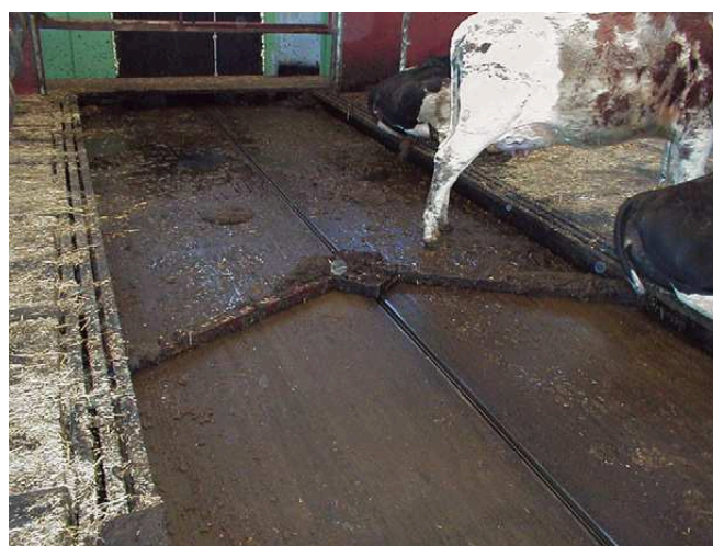
Figure 6-13 The central alley of this Swedish barn has a rubber floor and a mechanical scraper which ploughs both ways. Note that the back of the stall is fitted with slats which are also covered with rubber. (Courtesy of C Bergsten)
