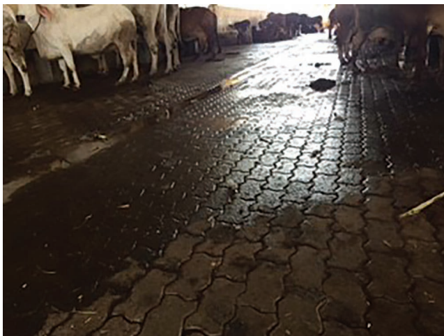
FIGURE 13.1 Concrete pave-block flooring at a gaushala in India.
