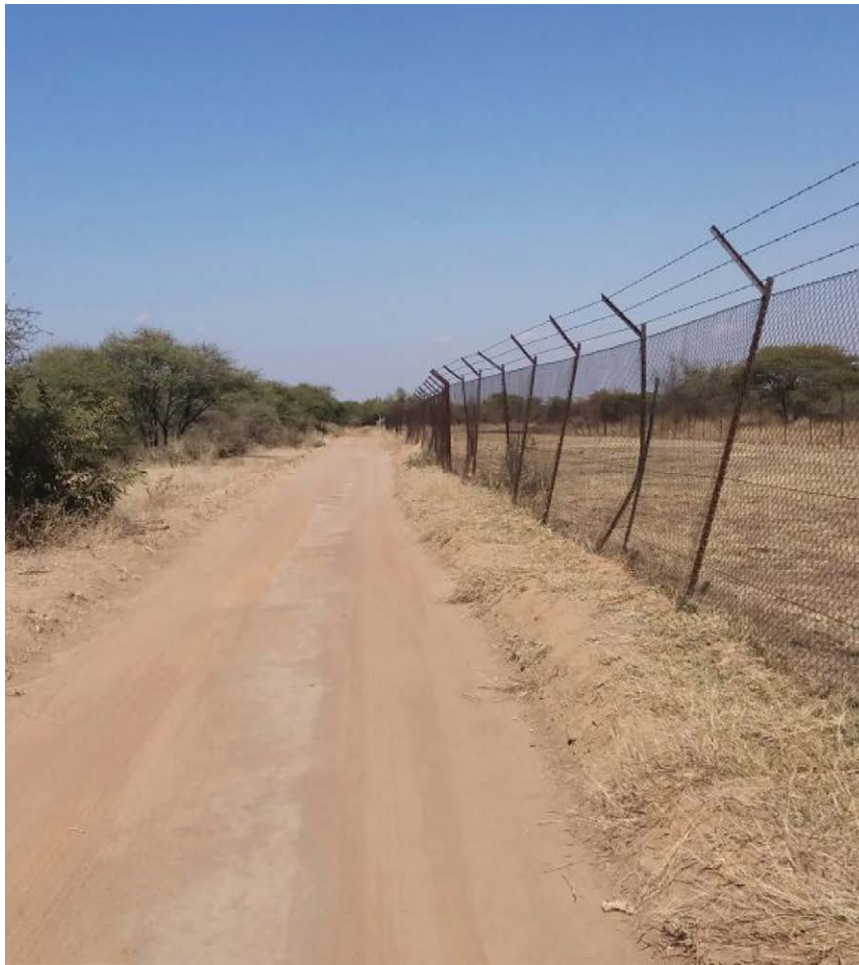
Fig. 4.6. The inner perimeter fence line facing into the reserve. The support post has been bent by the impact of impala or blesbok that have been run into the fence by caracal. These medium-sized cats have learned to use the fence as part of their hunting strategy. (Image credit: Charles Theron, used with permission.)
