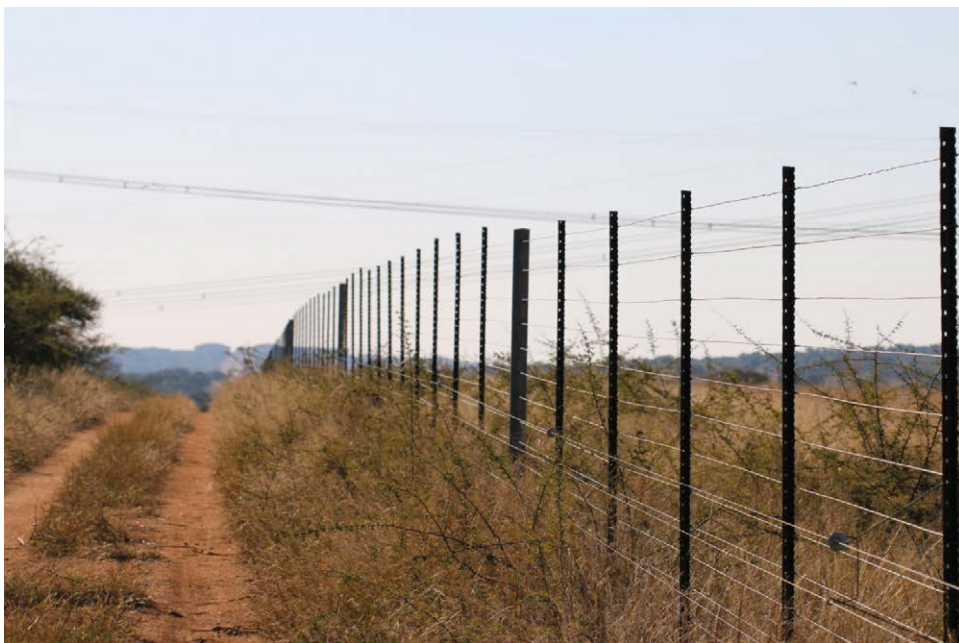
Fig. 4.1. The external perimeter fence of a wildlife reserve in South Africa. Multiple strands of wire are stretched between well-anchored posts to give a continuous boundary fence that keeps wildlife in and neighbouring cattle out. (Image credit: Adam G. Hart.)
