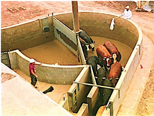
Fig. 6.6. Round crowd pen that has been filled half full. Note that the crowd gate is not pushed up tight against the animals. This design takes advantage of the natural behaviour of cattle and sheep to go back to where they came from. (From Grandin, T., 1998, in Gregory, N.G. (ed.) Animal Welfare and Meat Science . CAB International, Wallingford, UK.)
