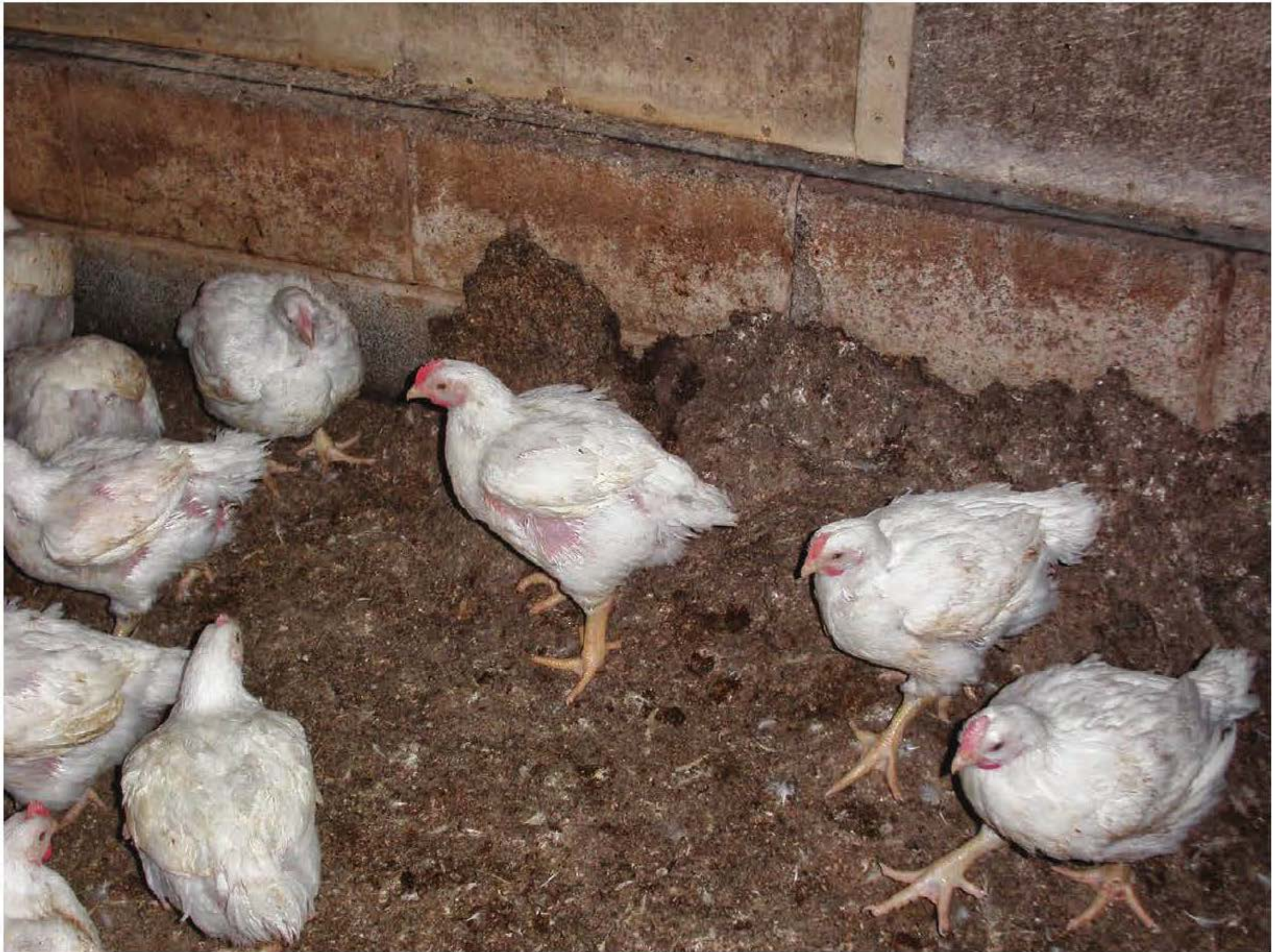
Figure 4.9 Poor cleaning in between flocks increases the risk of disease in the birds. In old buildings with cracked floors, non-smooth walls and wooden constructions, cleaning and disinfection between consecutive flocks can be quite difficult.
