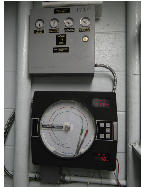
FIGURE 3.5 A monitoring station that tracks temperature, humidity, and air pressure and records temperature and humidity in an animal room.
