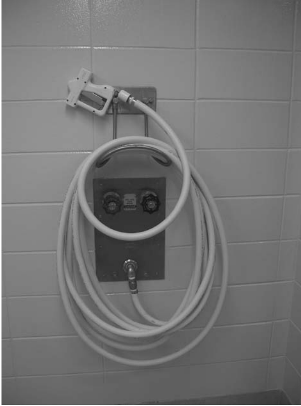
Figure 2.2 An ergonomic spray nozzle is used for spraying down dog kennels. These spray nozzles rotate 360 degrees about the long axis of the hose and reduce wrist fatigue during cleaning.
