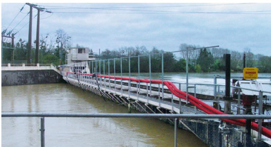
**Fig. 4.73** Angled screen (right) stretching across the former intake bay of the Baigts hydropower station on the Gave de Pau in France, as seen from the turbine intake (U. Schwevers)
