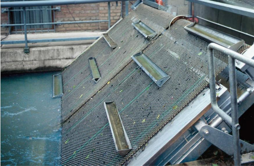
**Fig. 4.31** Former circulating screen with screwed-on troughs at the hydropower station on the German Elbbach in Hadamar (U. Schwevers)
