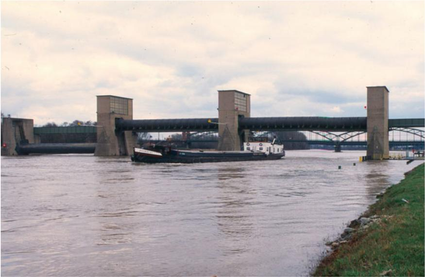
**Fig. 3.4** The weir in Kostheim on the German river Main at high water level; two of the three rollers have been lifted, clearing the way for ships (U. Schwevers)
