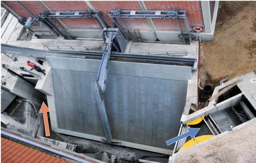
**Fig. 5.3** Bottom (orange arrow) and surface bypass (blue arrow) at the Netherlands hydropower station Roermond on the Rur (Ingenieurbüro Floecksmühle GmbH)
