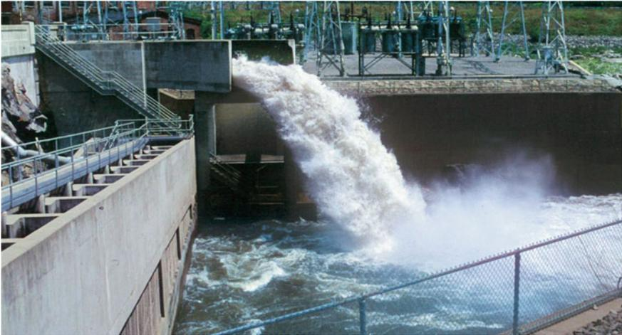
**Fig. 5.23** The outlet of the bypass at the Bellows Falls hydropower station on the Connecticut River (USA) is located approximately 9 m above the tailwater level (U. Schwevers)
