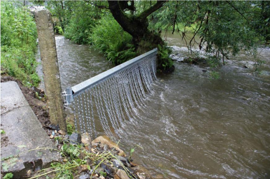
**Fig. 4.9** Hanging chain curtain of the Prossen hydropower station in the German Lachsbach (Archiv LfULG)
