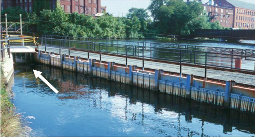
**Fig. 4.27** Louver in the headrace channel of a hydropower station at the Holyoke Dam on the Connecticut River (USA) (U. Schwevers)
