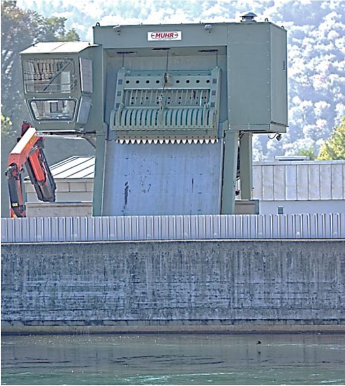
**Fig. 4.40** Wire rope cleaner for a screen with vertical bars (U. Schwevers)
