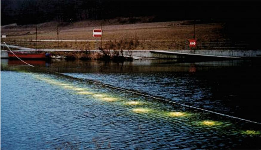
**Fig. 4.7** Light deterrent system at the German hydropower station in Dietfurt on the Altmühl river that proved to be ineffective (R. Hadderingh)
