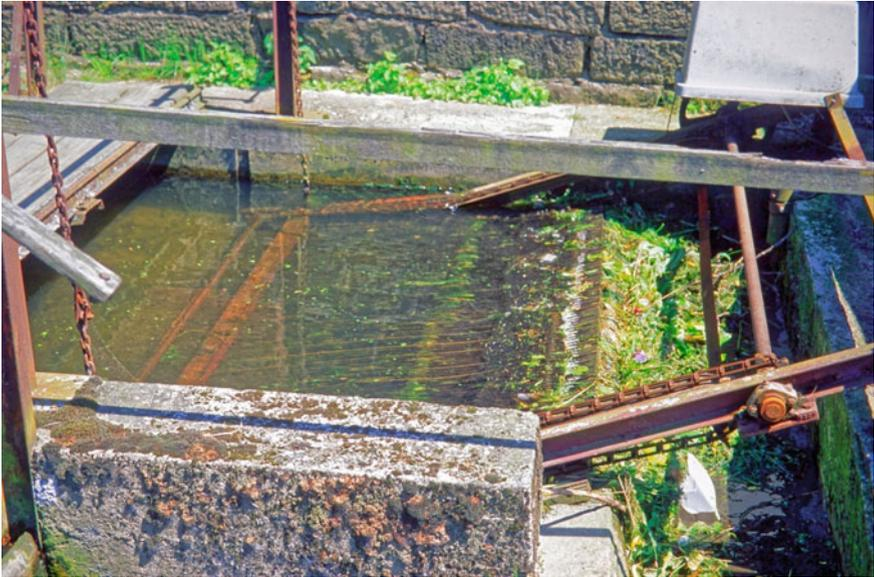
**Fig. 4.61** Flat inclined screen at a small historic hydropower stations in Germany (U. Schwevers)
