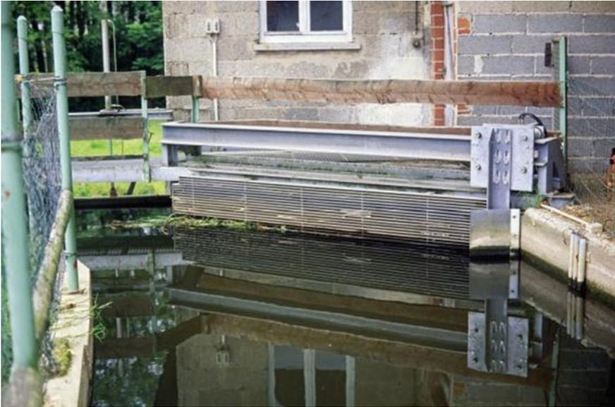
**Fig. 4.70** Angled screen with a flushing gate at its downstream end on the German river Döllbach (U. Schwevers)
