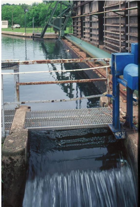
At the Röchlig hydropower station on the Swiss river Aare, a horizontal screen with a depth of 7.7 m was installed at the weir turbine ( $Q_{HP} = 40 \text{ m}^3/\text{s}$ ). According to the manufacturer, this construction depth is considered to represent the maximum size which is currently technically feasible, particularly because the screen cleaning system is pushing its limits as well.
