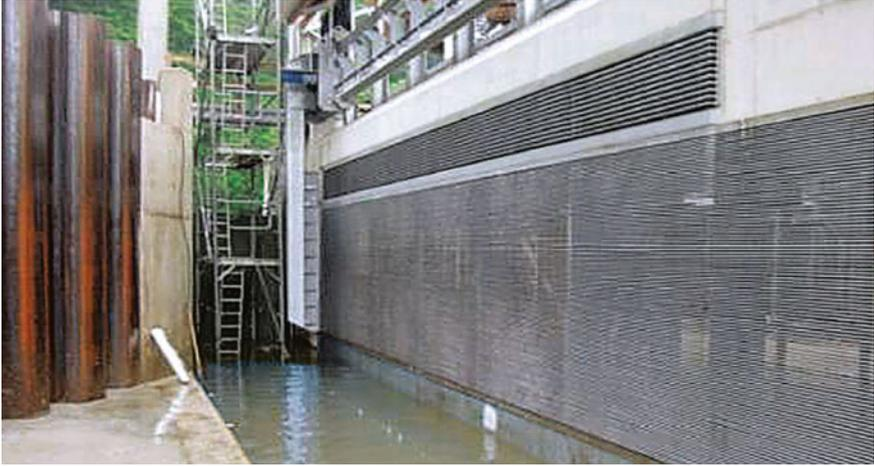
**Fig. 4.15** Angled screen with horizontal bars at the hydropower station Auer Kotten on the German river Wupper; discharge capacity  $Q_{HP} = 14 \text{ m}^3/\text{s}$ ; clear space  $s_R = 12 \text{ mm}$  (Ingenieurbüro Floecksmühle GmbH)
