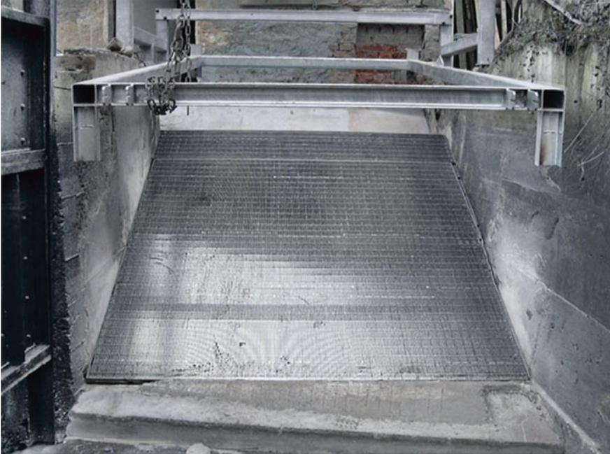
**Fig. 4.20** Inclined wedge wire screen with a clear space of  $s_R = 5$  mm in front of the intake of the Floecksmühle hydropower station on the Nette (Germany) (U. Schwevers)
