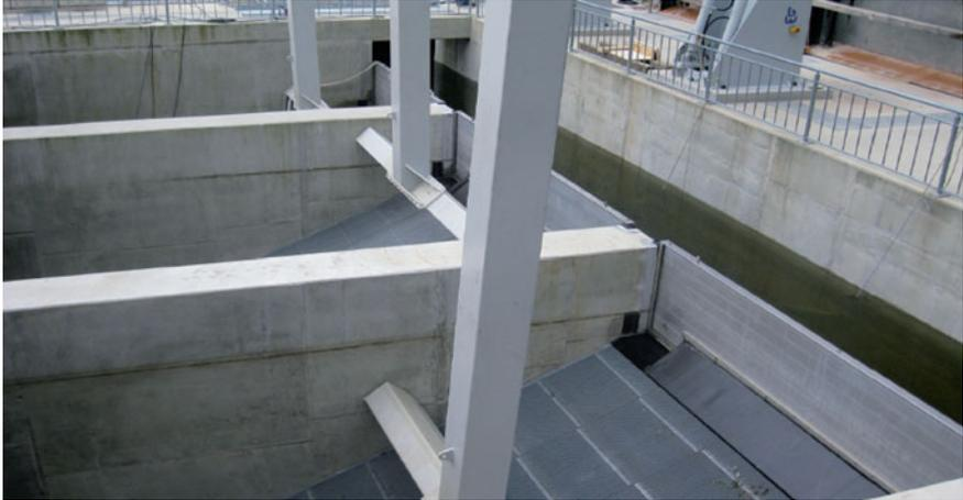
**Fig. 4.17** Inclined screens with a clear space of 10 mm with cleaning systems (Ingenieurbüro Floecksmühle GmbH)
