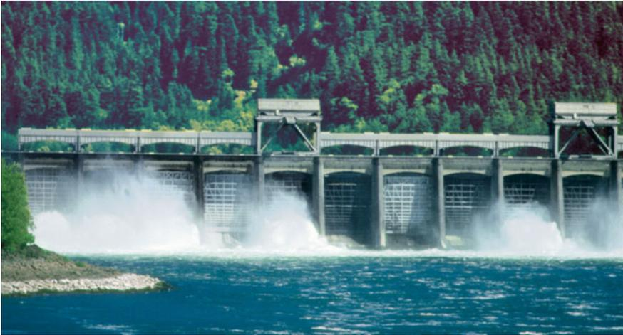
**Fig. 5.25** An additional weir discharge via sluice gates shaped like ski jumps supports the downstream migration of Pacific salmon smolts at the Bonneville Dam on the Columbia River (USA) (U. Schwevers)
