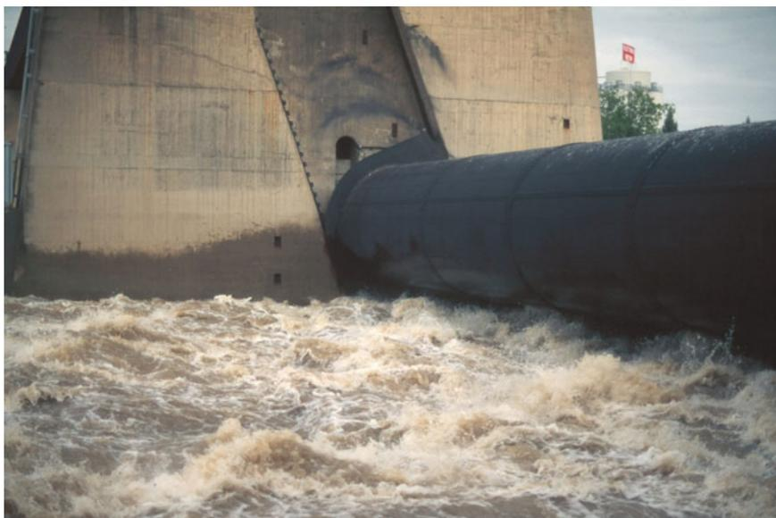
**Fig. 3.3** Undershot roller gate with high discharge (U. Schwevers)
