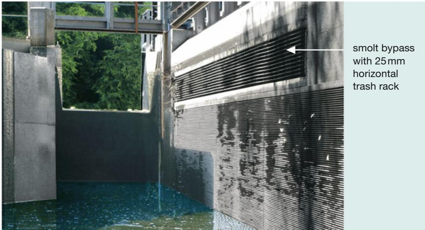
**Fig. 4.49** The smolt bypass (arrow) installed above the intake screen of the Auer Kotten power station on the Wupper is protected against floating debris by a 40 mm screen (U. Schwevers)
