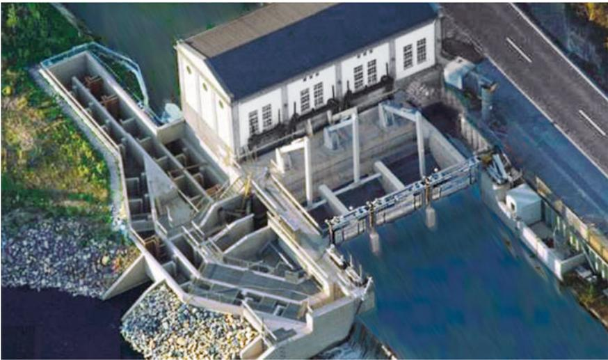
**Fig. 4.16** Top view on Unkelmühle hydropower station on the German river Sieg; discharge capacity  $Q_{HP} = 28 \text{ m}^3/\text{s}$ ; intake area with three inclined screen systems (Fig. 4.17) (Wikipedia)
