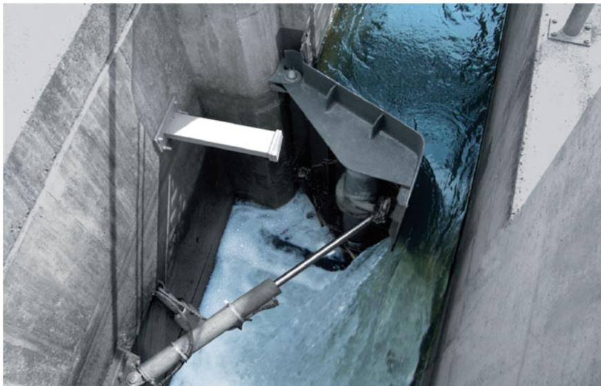
**Fig. 4.72** Bypass with a swing gate at the Planena hydropower station
