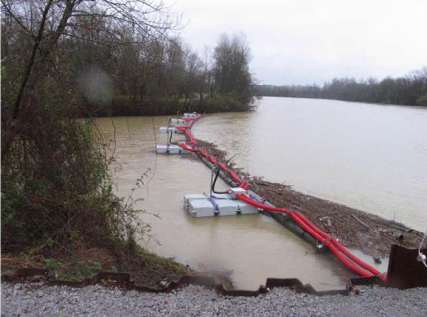
**Fig. 4.6** Infrasound system in the headrace channel of the Biron hydropower station on the Gave de Pau (France) (U. Schwevers)
