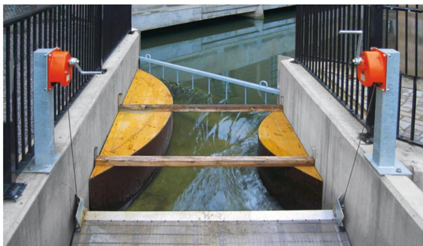
**Fig. 5.22** Entrance of the salmon bypass at the hydropower plant on the Rur (Netherlands) with temporary inserts for optimizing the flow conditions (Ingenieurbüro Floecksmühle GmbH)
