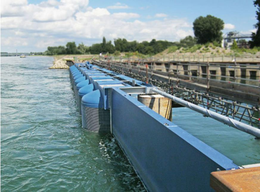
**Fig. 4.37** Cooling water intake of the German Rhine Port steam power plant in Karlsruhe with a RO-TEC™ screen consisting of 12 drums (Erhard Muhr GmbH)
