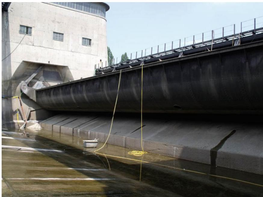
**Fig. 3.7** Drained center weir field of the weir in Offenbach on the German Main; the fixed weir sill on which the movable fish-belly flap rests rises above the concrete floor (U. Schwevers)
