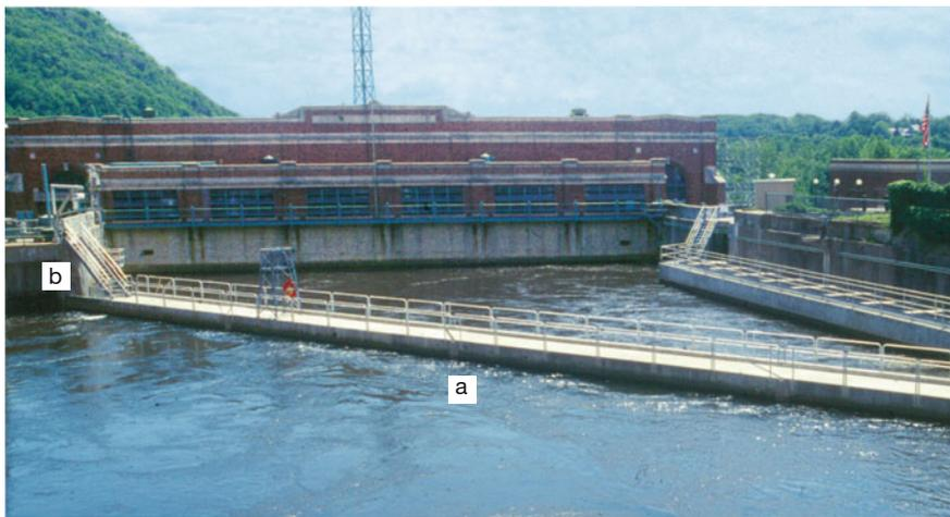
**Fig. 4.82** Baffle in front of the intake of the Bellows Falls hydropower station guides descending salmon smolts towards a bypass (Ingenieurbüro Floecksmühle GmbH)
