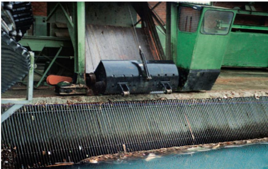
**Fig. 4.11** Conventional bar rack with screen cleaning system (U. Schwevers)
