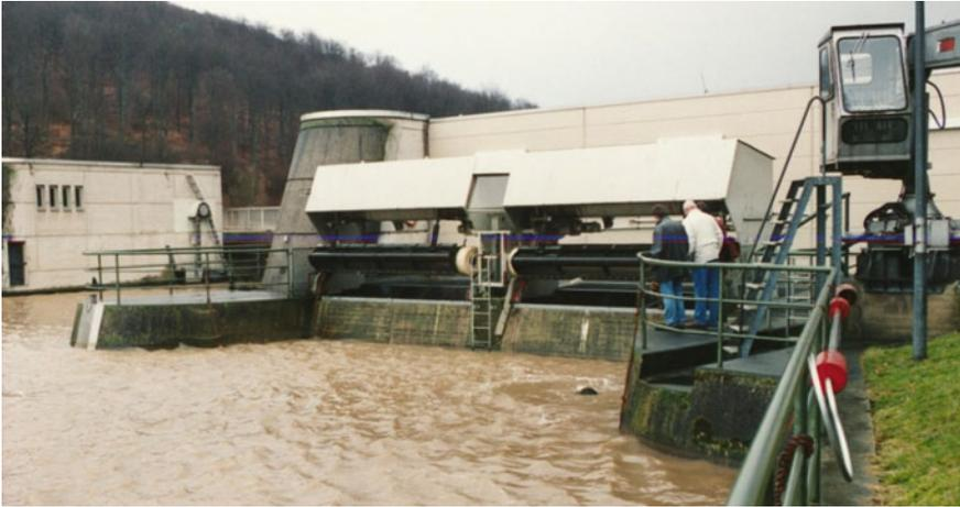
**Fig. 4.52** The Wahnhausen hydropower station on the Fulda which was retrofitted with a 20 mm screen in 1990 (U. Schwevers)
