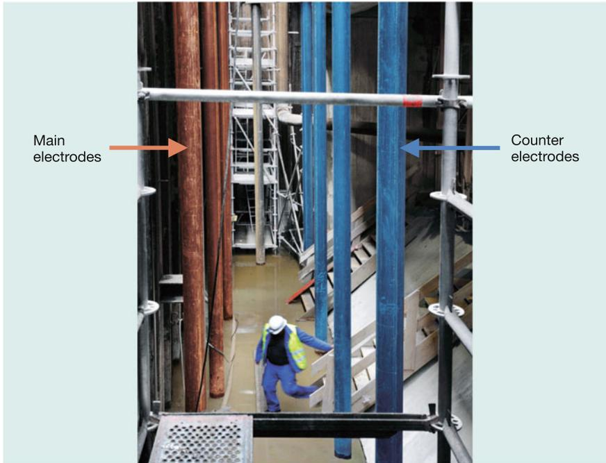
**Fig. 4.3** Electrodes of the electric deterrent system at the water intake structures of a thermal power station under construction (U. Schwevers)
