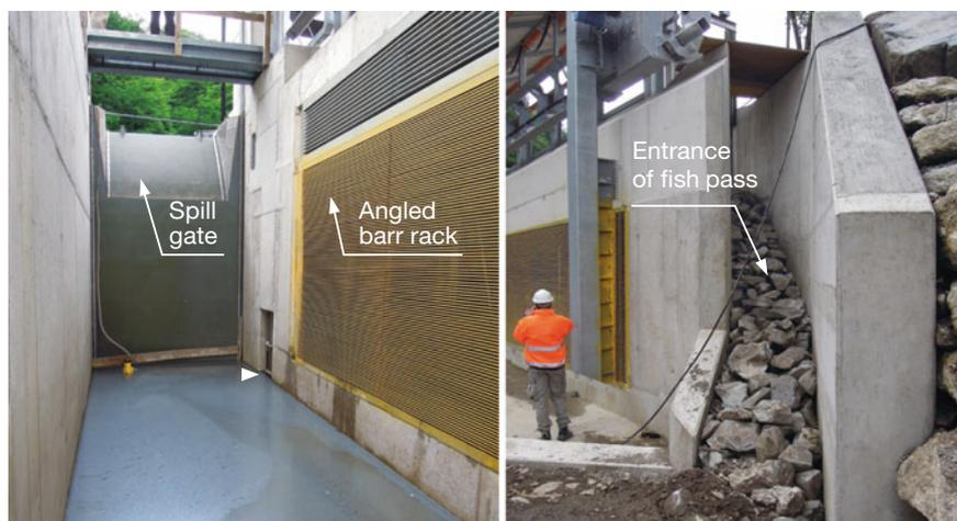
**Fig. 4.79** Angled screen of the German Auer Kotten hydropower station on the river Wupper with three bypasses and a spill, resp. flushing gate at the downstream end of the screen (left) and the entrance of the fish pass at the upstream end (right) (Ingenieurbüroe Floeckmühle GmbH)
