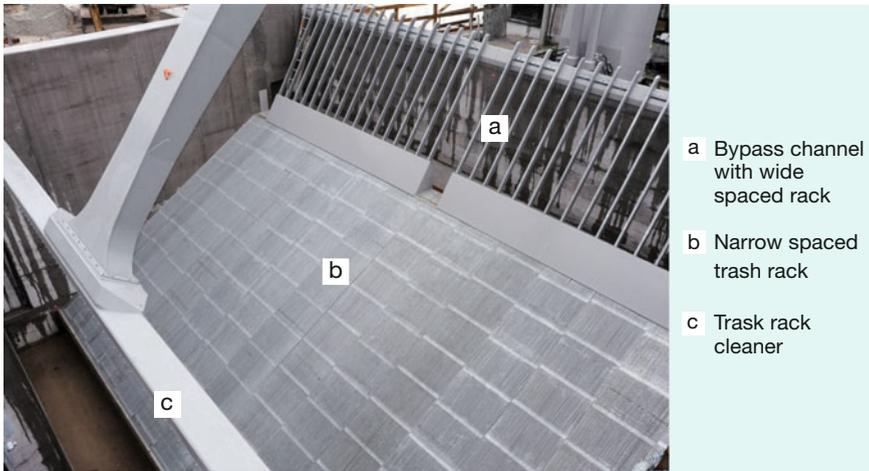
**Fig. 4.62** German hydropower station Willstätt on the river Kinzig with an inclined screen with vertical bar orientation,  $s_R = 10$  mm, inclination  $\alpha = 30^\circ$ ,  $Q_{HP} = 25$  m<sup>3</sup>/s (Ingenieurbüro Floecksmühle GmbH)
