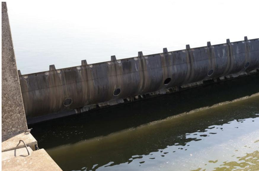
**Fig. 3.6** Fish-belly flap with flow splitters along the upper edge (U. Schwevers)
