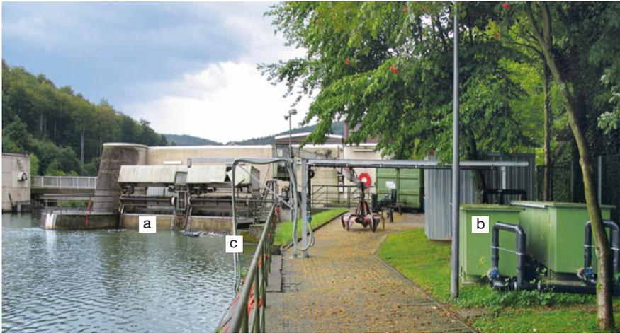
**Fig. 7.4** MIGROMAT™ at the Wahnhausen hydropower station on the river Fulda (Germany) with the turbine intake in the background (a). Two green tanks with eels (b) are watered by submersible pumps on a crossbar (c) (U. Schwevers)
