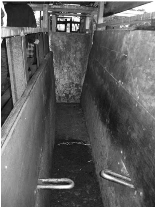
Figure 27. A V-shaped race prevents animals turning around. This race also has backing bars protruding into the race. As the cattle push on these they swing forward, springing back into place behind the animal, preventing the animal from backing down the race.
