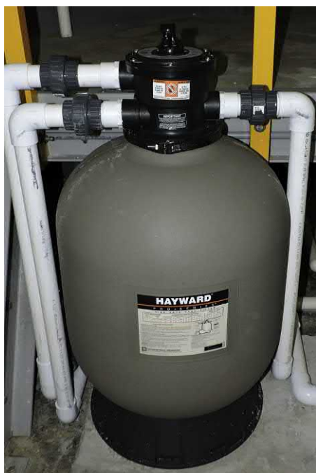
FIGURE 30.3 A rapid sand filter used as a mechanical filter. Picture courtesy of McWane Science Center Birmingham AL.
