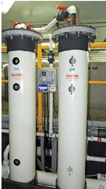
FIGURE 30.6 Two fluidized sand filters. Picture courtesy of McWane Science Center.
