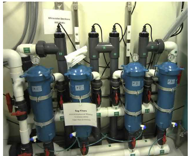
FIGURE 30.5 Pressurized bag filters to provide mechanical filtration prior to ultraviolet (UV) disinfection. Note the pressure gauges on top of the canisters to notify technicians that the bags need to be cleaned or changed. Note the UV disinfection units behind the pressurized bag filters. Picture courtesy of The University of Alabama at Birmingham.
