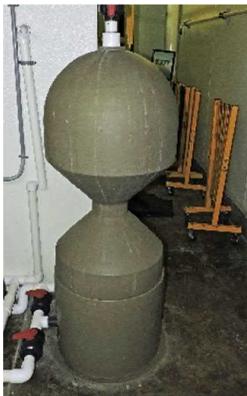
FIGURE 30.4 A floating bead filter used as a biological filter. Picture courtesy of McWane Science Center Birmingham, AL.
