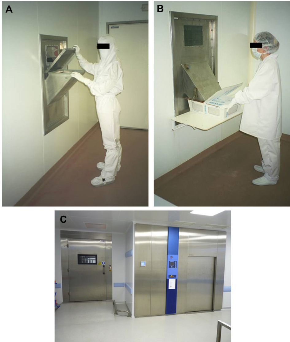
Figure 4.6.3 Full-barrier room. A. Barrier area fittings: rodent shipping chute with communication window. (C) Left: Breeding barrier side. Right: Shipping room side (photo credit: Janvier). B. Barrier area fittings. Left: hydrogen peroxide chamber. Right: Steam autoclave (photo credit: Sanofi R&D).
