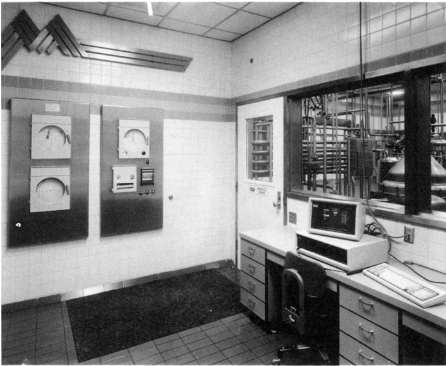
Fig. 2. Computer control room showing a desk-top personal computer used with a programmable logic controller for formulating mixes, assembling mixes, operating all processing equipment in the plant and controlling the cleaning and sanitising of equipment and pipe lines. The sub-panels on the wall at the left are those instruments required (in the US) for legal control. (Reproduced by courtesy of Seiberling Associates, Inc.)
