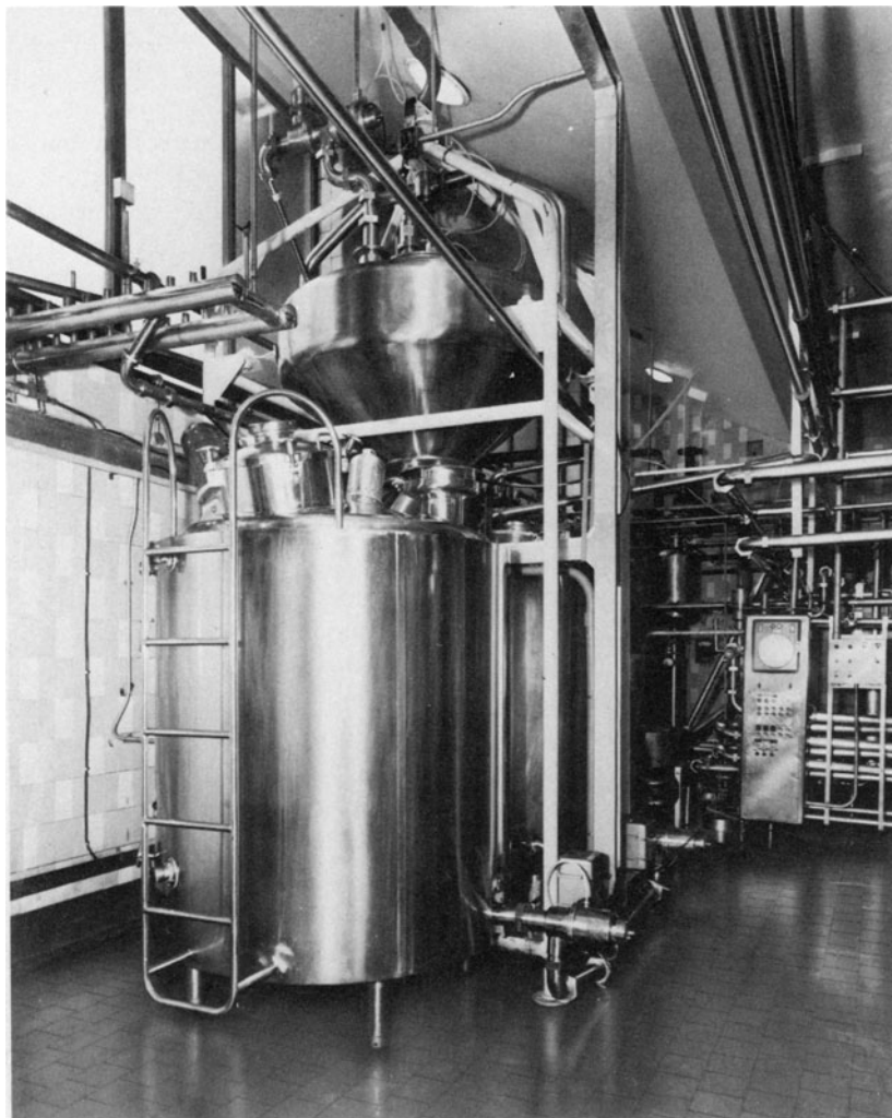
Fig. 1. Automated mix batching system. The weigh tank with its load cell is suspended above two blending tanks. After each ingredient is weighed, the control system indicates or records the weight and opens a valve to allow the ingredient to flow into one or the other blending tank. After a batch is completed, the next is weighed and dropped into the other blending tank. (Reproduced by courtesy of APV International, Ltd.)
