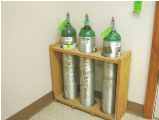
FIGURE 20-9 Oxygen tanks need to be properly secured.
