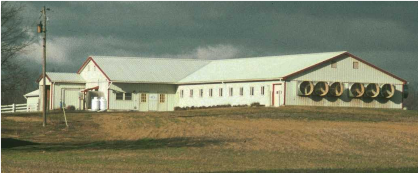
FIGURE 15-5 Barn equipped with tunnel ventilation.
