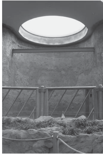
Figure 6.11 The provision of light to inside enclosures can be difficult to achieve because many materials prevent light penetration, especially at UV wavelengths. In this elephant exhibit at Duisburg Zoo, great efforts were made to increase the light levels and a custom-made polymer was fitted to allow UV light penetration. (Photographs: Vicky Melfi)
