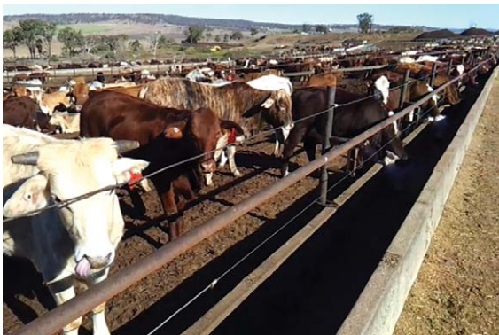
Fig. 11.3. Cattle feedlot built into the side of a hill to aid drainage.
