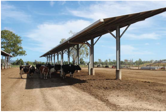
Fig. 8.7. Angled shade for dairy cows in Queensland, Australia, over a lying pad with woodchip base covered with compost on top, scarified regularly to provide a comfortable lying area.
