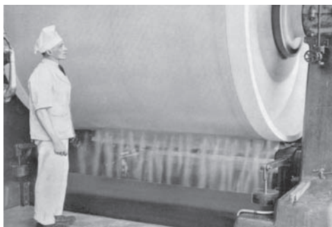
Figure 6.6 Chill drum. Source: Robinson and Rajah (2002).
