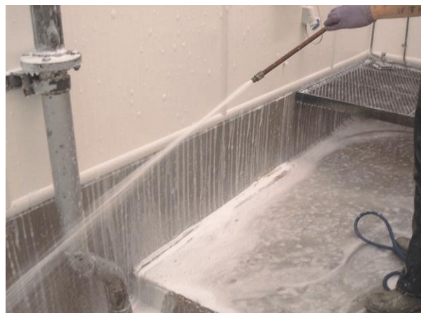
Figure 3 Use of QACs foam products for disinfection of food processing premises.
