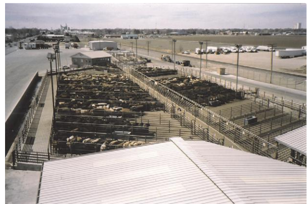
Figure 3 Herringbone stockyard/lairage with long narrow pens. Cattle enter through one end and exit through the other end. The correct angle for the pens is 60–80°.
