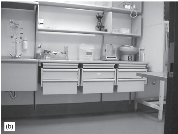
Fig. 15-14 Animal procedure area in a large animal cubicle room showing: (a) the wall-mounted sink and examination table, and the ceiling-mounted hose reel; (b) the wall-mounted counter and open design case work leaving the floor open for cleaning and reducing harborage sites for insects and vermin.
