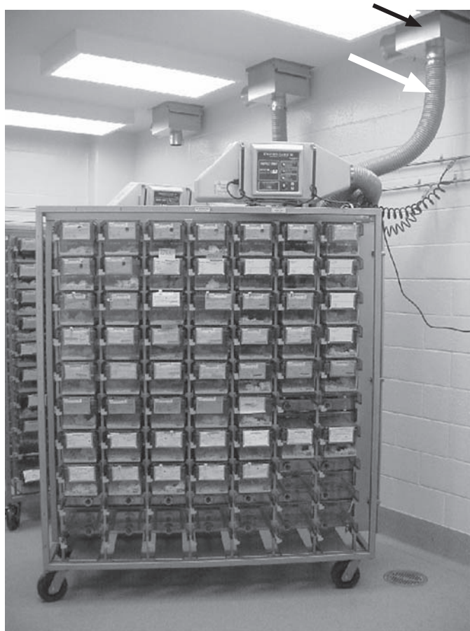
Fig. 12-7 Mouse individually ventilated cage effluent ducted to the building exhaust (white arrow) through a transition device/damper mechanism (black arrow).
