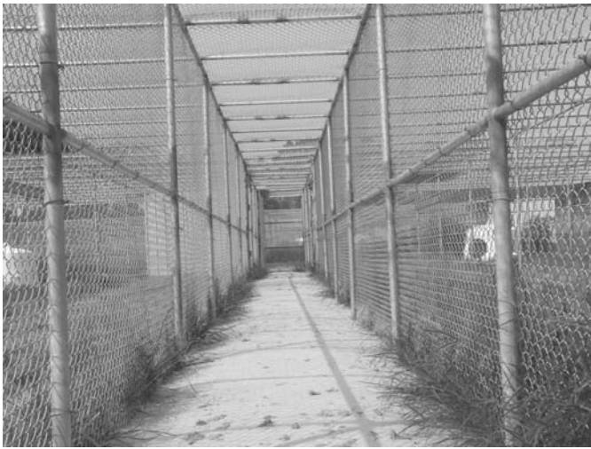
Fig. 21-24 Berm for separation of enclosures in divided field cages. Berms are used to separate enclosures that are in close proximity by directing wastewater runoff away from adjoining enclosures and preventing contact between animals. The photograph shows a concrete berm that is within a divided field cage and is 5 feet wide.
