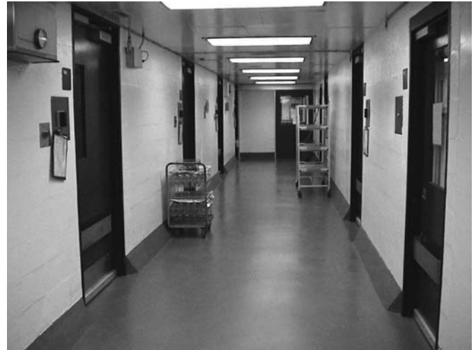
Fig. 9-5 Picture of an animal facility corridor illustrating 6" × 6" sloped bases designed to protect the walls. The bottle cart and cage rack show how the base serves to protect the wall. They also show how the low-mounted crash rail in Figure 9-3 would effectively protect the wall from being hit by either short or tall carts.
