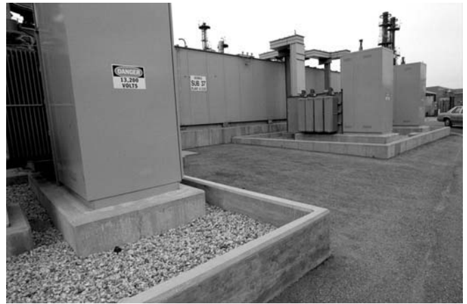
Fig. 14-1 Electrical substations have been raised by placing them on concrete slabs and surrounding them with concrete curbs to protect them from flood damage.
