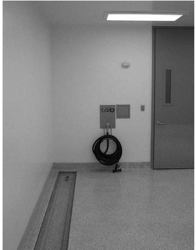
Fig. 22-4 Trench drain along the side wall of an animal room equipped with a central rim flush floor drain (outside bottom of photograph) and water jets at both ends to flush waste towards the drain. A wall-mounted hose bib is available in the room.
