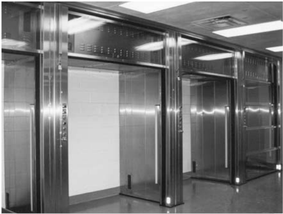
Fig. 15-22 Prefabricated isolation cubicles are shown with stainless-steel divider walls. These cubicles include individual, local air-control packages with high supply and low return. Cubicles typically employ the facilities wall for the back side of the cubicle, as seen here.
