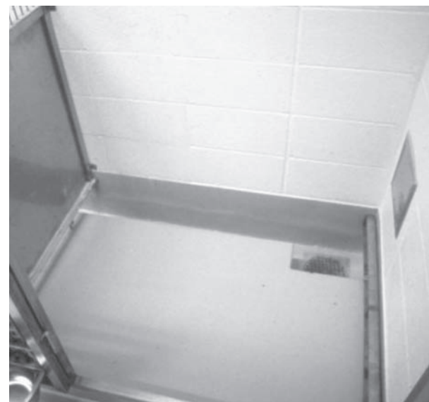
Fig. 18-5 A room equipped with free-standing dog runs: (a) the runs; (b) the trench drain at the back of a run. This room can easily be converted to another use by disassembling the runs, moving them to storage, and moving other caging equipment into the room.
