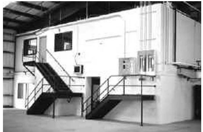
Fig. 14-4 Utilities components and switches can be protected from flood damage by elevating them. Platforms can be attached to allow maintenance personnel to easily access these components.
