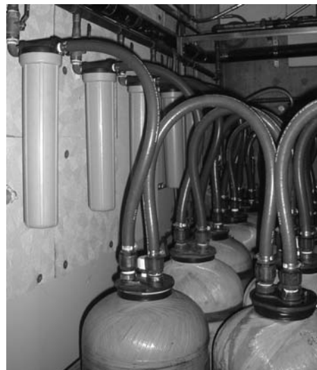
Fig. 23-2 Primary filtration system designed to remove chlorine and chloramines. In this photograph, water entering from the left is piped through five rows of activated charcoal filtration canisters (left arrow) and roughening filters (right arrow) before entering the aquatic facility.
