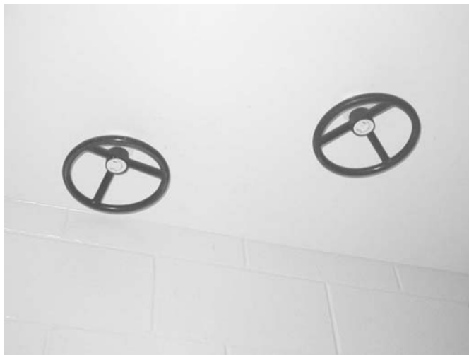
Fig. 25-6 Remote air supply/exhaust damper controls.
