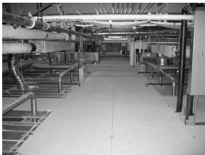
Fig. 13-3 Example of partial interstitial space with walkways (Washington University School of Medicine, St Louis, Missouri).
