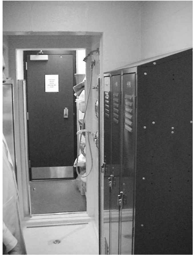
Fig. 24-3 (Continued) (b) Photograph of such a dressing/shower room looking into the entry portion with lockers. Note the closed shower door. (c) The same view as (b) with the shower doors open, looking through to the door leading into the containment area.
