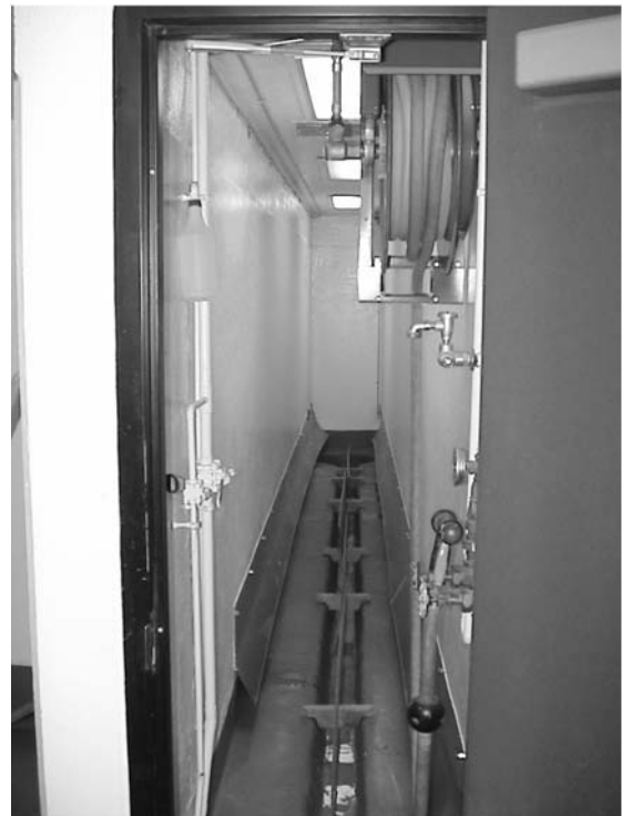
Fig. 15-15 View of a 30"-wide service area for large animal cubicle rooms on both sides showing the drain trough running the length of the room and the stainless steel flashing attached to the walls that helps to direct water and waste from the adjacent pens on both sides into the trough. Also shown are the hose reel, the vertical splash panel suspended in the center of and running the length of the trough to prevent water from splashing across the trough into the next room, and the lever-controlled ball valve on the left that controls the water running down the drain trough and in the flush drain at the other end of the trough.
