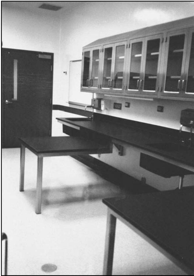
Fig. 19-5 (b) Diagnostic laboratory. Upper stainless steel cabinetry, wall-mounted work-counter space, and two-microscope counter surfaces are shown. Note that none of the casework extends to the finished floor, which facilitates cleaning. (c) Diagnostic laboratory. This is Figure 19-5(b) from a different angle.
