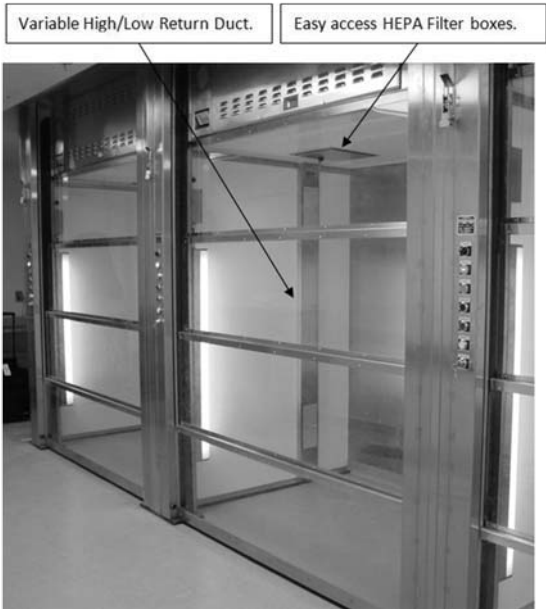
Fig. 15-23 Prefabricated cubicles are shown with SIP (structural insulated panels) divider walls. These cubicles include individual air-control packages with high supply and variable high/low returns. Duct covers allow the user to “select” the type of return air (high or low) depending on the specific science demands. Note these cubicles are extra deep and allow more space for procedures inside the protected cubicle space.
