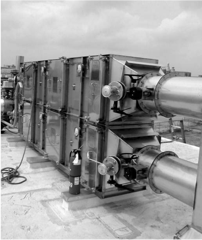
Fig. 34-5 Redundant bag-in/bag-out HEPA filters.
