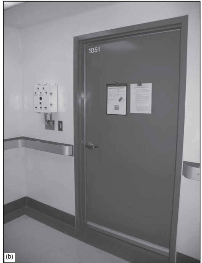
Fig. 19-4 (b) Entrance to gas cylinder storage room. This room is conveniently located outside of the surgery suite and easily accessible by delivery personnel. The alarm adjacent to the door is located in an area of high traffic and visibility, to alert personnel when a gas supply cylinder has been depleted and the manifold needs to be switched to obtain gas from a full cylinder or cylinder replacement is necessary.
