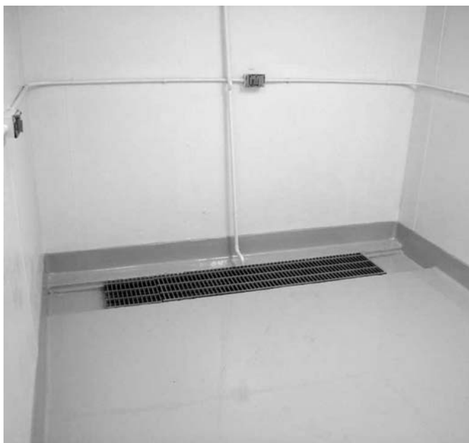
Fig. 23-3 Trough floor drain shown with fiberglass grate cover (end pieces removed) along the back wall of a small aquatic room. Electrical outlets are located on the wall 3–4 feet above the floor.
