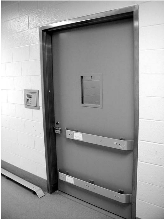
Fig. 4-26 Animal room door mock-up in progress shows hardware and vision panel details.
