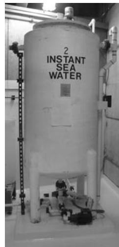
Fig. 23-1 Holding tanks for natural and artificial sea water. In this facility, marine water is exclusively carried in polyvinyl chloride (PVC) pipes and all plumbing is exteriorized.
