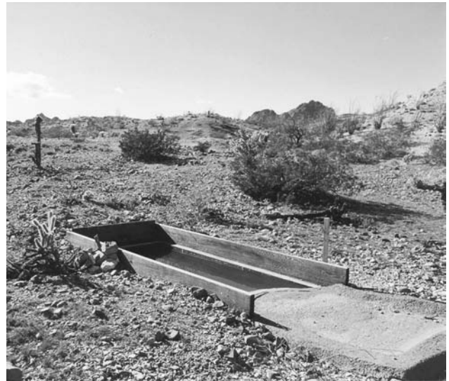
Fig. 27.7. Underground guzzlers are nearly invisible to humans that are more than a few meters away, making them especially useful in designated wilderness areas. Guzzler design by Lesicka and Hervert (1994).
