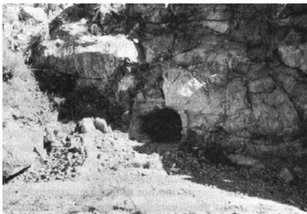
Fig. 27.4. An adit is a short tunnel that has been blasted into solid rock to store water for wildlife. The entrance to the adit must be at the same elevation as the bottom of the wash in which it is located.
