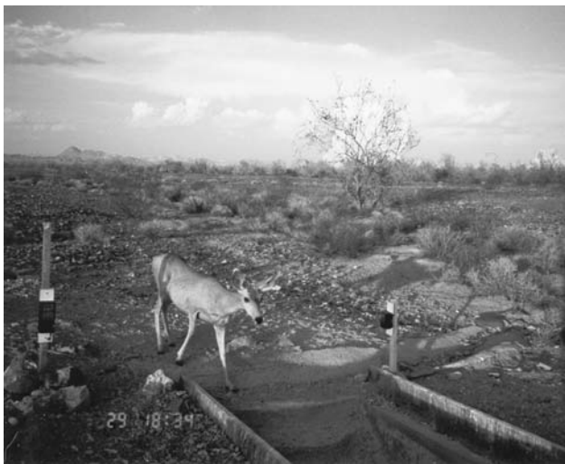
Fig. 27.5. Contemporary underground guzzlers store up to 40,000 L of water and have no moving parts. Wildlife walks down a ramp to reach stored water. Guzzler design by Lesicka and Hervert (1994).
