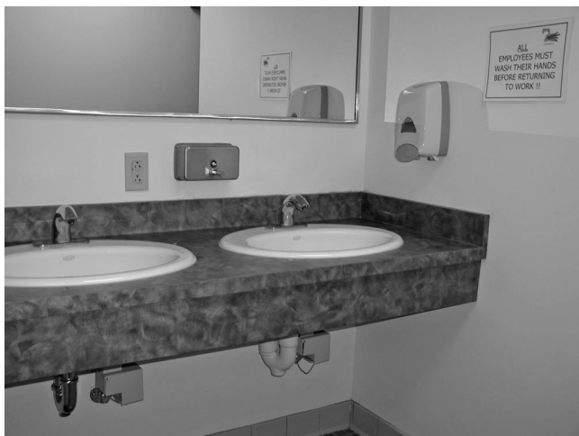
FIG. 2 Sensor-activated sink, liquid soap dispenser, and posted reminder for employees to wash hands after using the bathroom.
