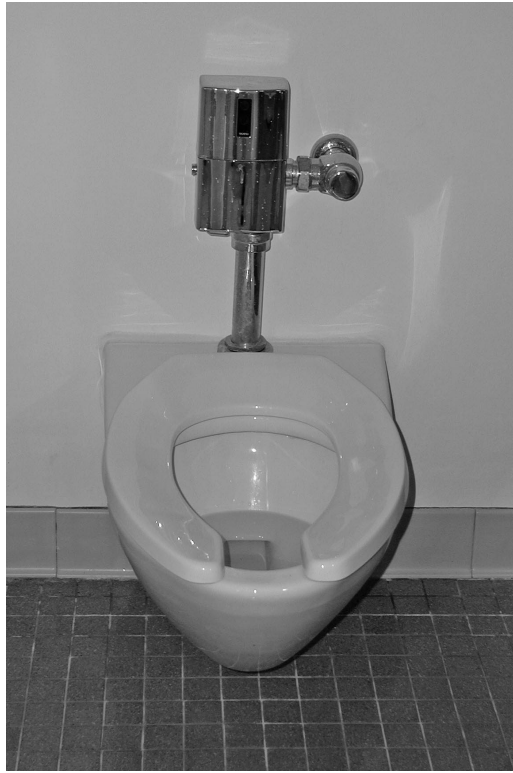
FIG. 3 Self-flushing toilet (infrared sensor) installed in employees' bathroom to minimize contamination.
